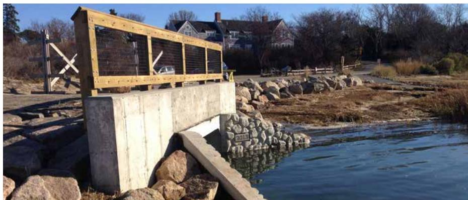
Freemans Pond Restoration project, completed in 2013, installed a new culvert to improve tidal flow, site drainage and water quality to 21 acres of coastal wetlands.
