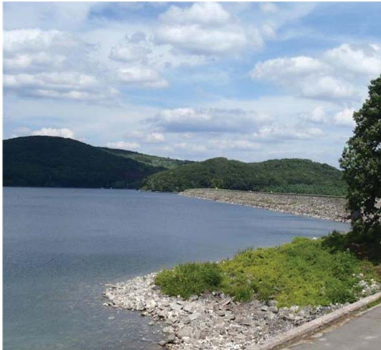
Just to the east of the Administration Complex one can see the Winsor Dam, an earthen structure with stone facing that holds back the 412 billion gallon Quabbin Reservoir (left). The Quabbin Observation Tower (right) situated at the summit of Great Quabbin Hill, is an 84' tower that was completed in 1941 for use as a fire watch tower as well as for public viewing. Accessed via Rt. 9, recent rehabilitation has made it ready for the fall "leaf peeping" season.
