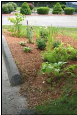
Installing rain gardens along streets to collect runoff is a common retrofit.
