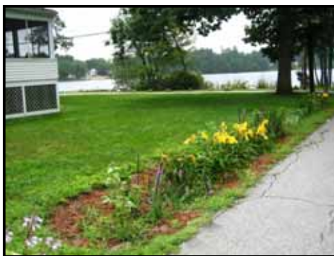
Rain gardens on Silver Lake Ave. and Dexter St. collect rain water that flows off the street and allow it to slowly soak into the ground.
