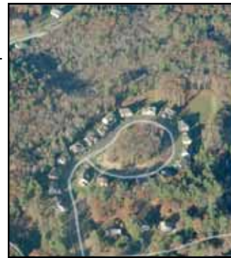
New developments can save open space by clustering homes and minimizing paved surfaces.
