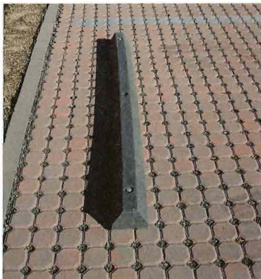
Tire stops made of recycled plastic were included at each parking space.
