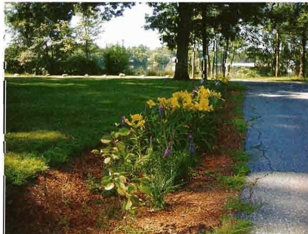
At sites at which lawns were higher than the roadway, rain gardens were redesigned in a longer, narrower fashion to create a gradual slope from the rain garden up to the lawn area.
