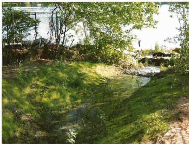
Two vegetated swales were designed and installed to replace a storm-water outfall that discharged directly to Silver Lake.
