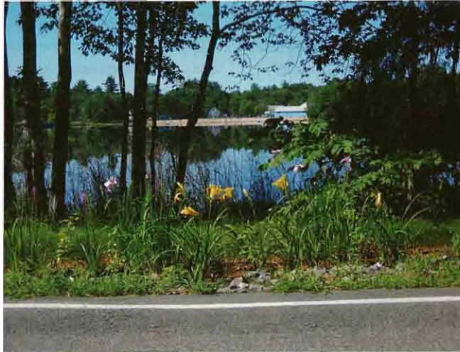
Several rain gardens constructed throughout the residential project area are expected to improve the quality of storm-water runoff and facilitate infiltration to recharge groundwater.
