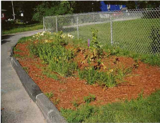
Twelve rain gardens were constructed on right-of-way owned by the Town of Wilmington in the Silver Lake watershed. In choosing the garden sites, preference was given to locations that would make it easy to convey runoff from the street.
