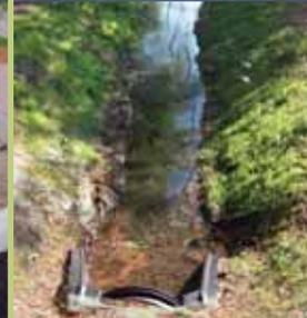
On Silver Lake Ave. and Dexter St., across the lake from the town beach, **rain gardens** and permeable pavers were installed along the street. Rainwater from roofs, driveways, and the street will drain to these areas, where it will be filtered and recharged to the ground.
