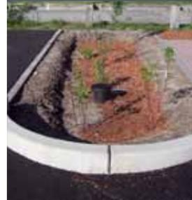
Stormwater pipes at either end of the beach have been replaced by **planted swales**, which filter and reduce runoff, prevent erosion, and discourage geese from gathering.
