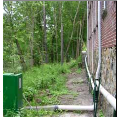
Water quality monitoring station below the green roof— Photo: DCR
