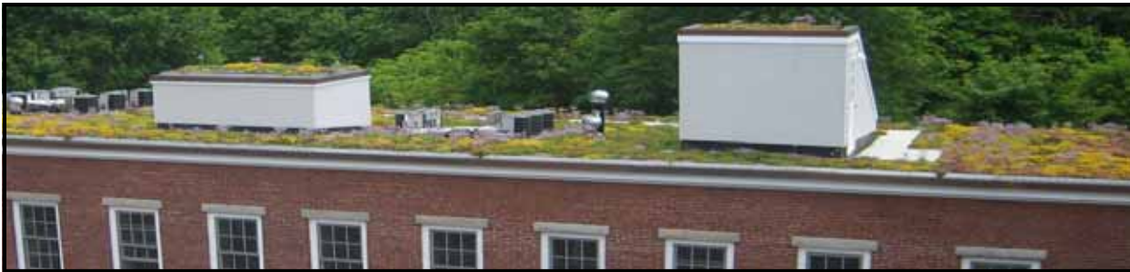
The case-study green roof was constructed in September 2006 on an existing roof (top) and is home to at least 10 species of flowering plants (bottom). The roof area is 3,000 ft 2 and the weight is 20 lbs. per ft 2 (saturated).
