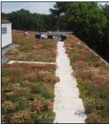
The case-study green roof was constructed in September 2006 on an existing roof (top) and is home to at least 10 species of flowering plants (bottom). The roof area is 3,000 ft 2 and the weight is 20 lbs. per ft 2 (saturated).
