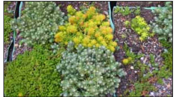
Dominated by succulent Sedums, green roofs need very little water or fertilizer and can survive temperature extremes.
