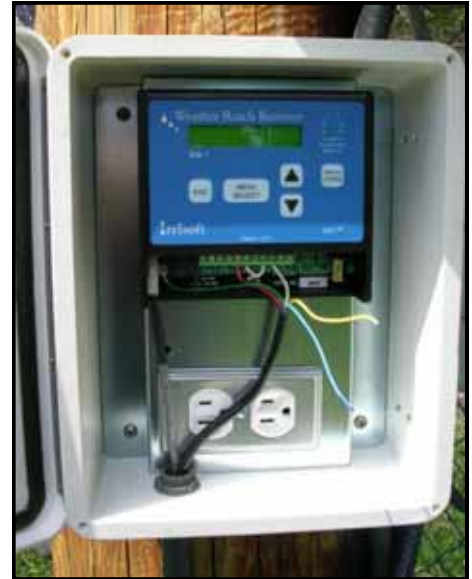
Weather-based irrigation controllers automatically control irrigation systems in response to rainfall so water is not wasted.
