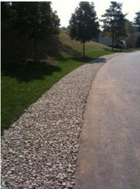
Road edge after grass pavers were replaced with river stone
