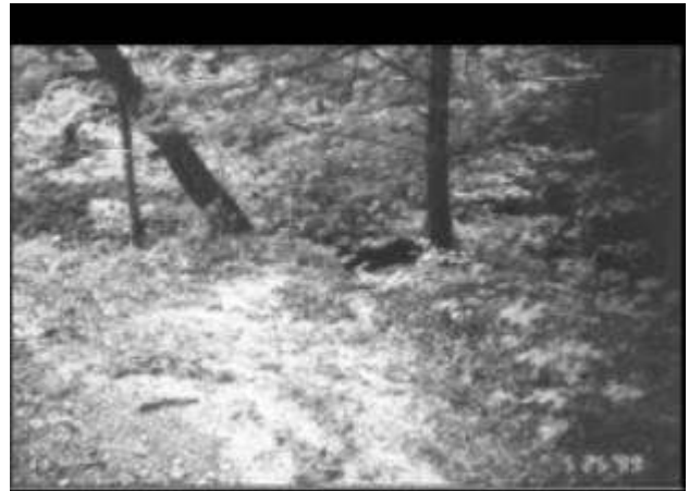
2. Erosion from the road surface and roadside bank were accumulating near and washing into the river.
