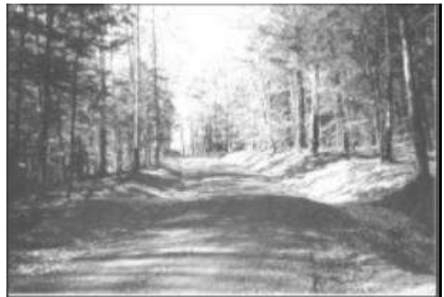
4. Completed road project.
