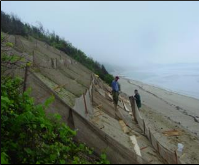
Lightweight, natural-fiber, erosion-control fabric was installed on this bank to protect the plants from wind until the roots could get established. Boards were placed on top of wooden stakes to provide access during construction, which minimized impacts to the bank from foot traffic. The photo on the right was taken one year after planting. (Photos: New England Environmental, Inc.)
