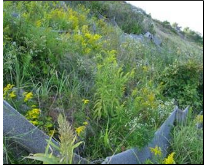
Lightweight, natural-fiber, erosion-control fabric was installed on this bank to protect the plants from wind until the roots could get established. Boards were placed on top of wooden stakes to provide access during construction, which minimized impacts to the bank from foot traffic. The photo on the right was taken one year after planting. (Photos: New England Environmental, Inc.)
