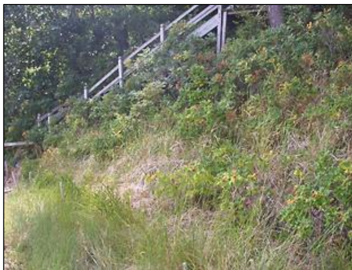
A variety of salt-tolerant vegetation was planted on the face of this bank to stabilize fill added to address bank erosion. (Photo: CZM)
