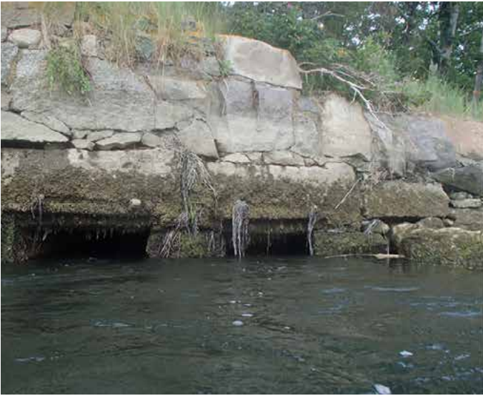
Undersized culverts (left) prior to being replaced with new bridge (right)
