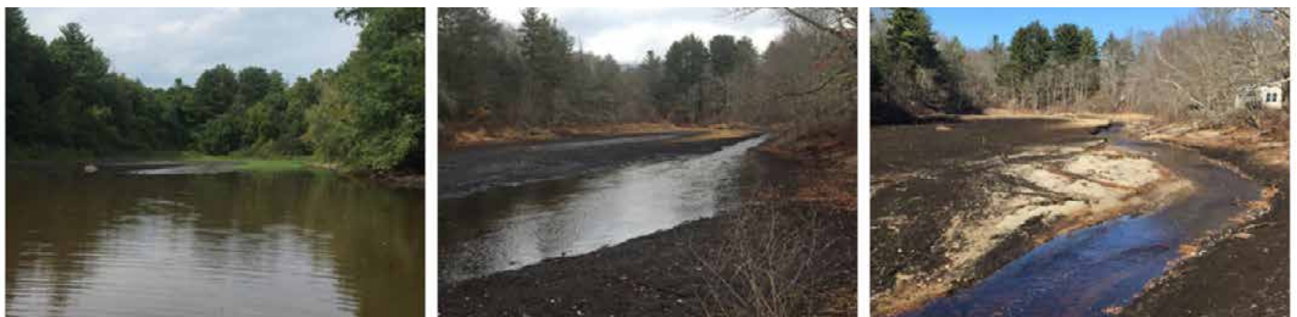
Impoundment behind Tack Factory Pond before removal (left), after removal in January (middle) and in March (right)
