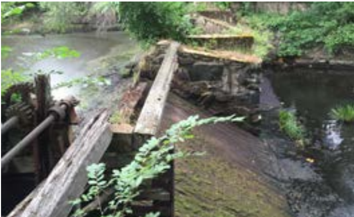
High Street Dam in Bridgewater
