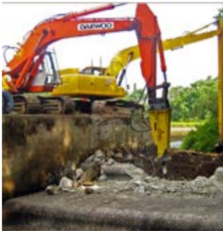
Start of Hopewell Dam Removal
