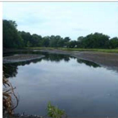
During Dam Removal (2012)
