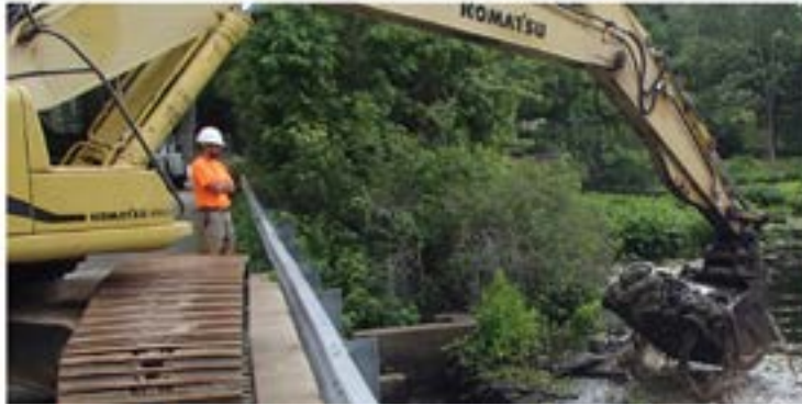
The Hunters Pond Dam removal in process.
