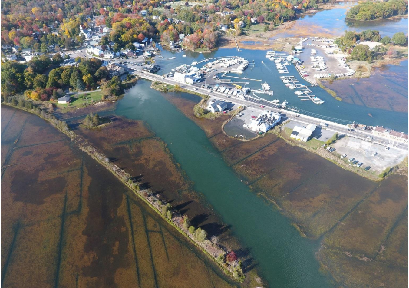
Essex Causeway/Main Street and businesses showing inundation from the Essex River. Photo credit: Abby Manzi, DeRosa Environmental
