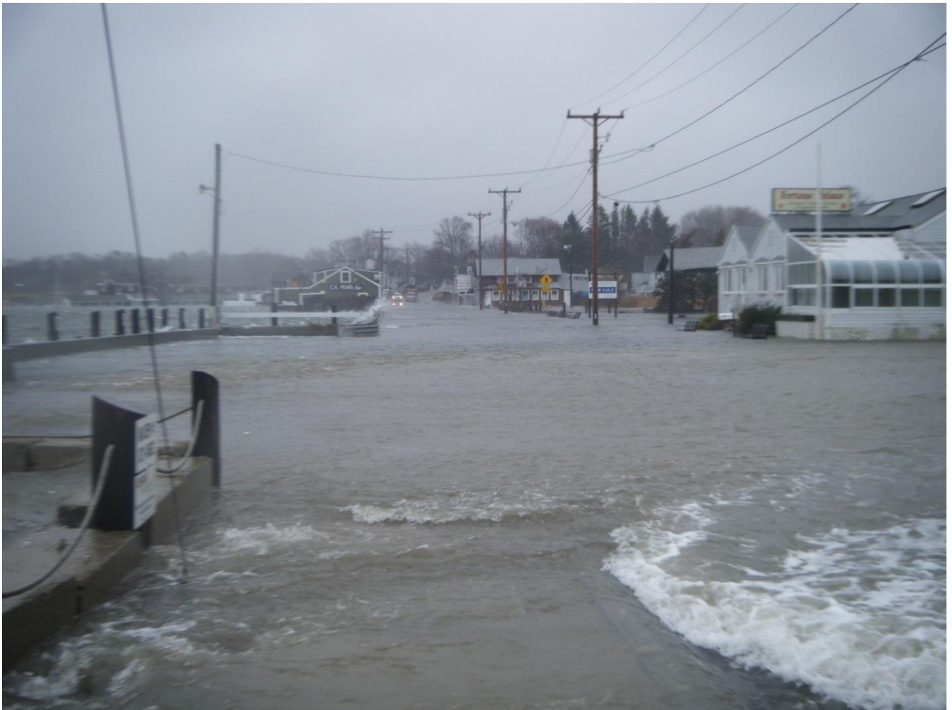
Route 133/Main Street "Essex Causeway", Essex, MA. Winter storm and tidal flooding, March 2, 2018
