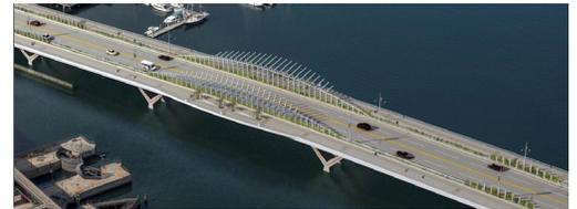
The structure will also improve water flow and conditions for boaters by reducing the number of piers in the water from 12 to 5, and widening the navigation channel to 141'. The new bridge is estimated to cost \$177 million.
