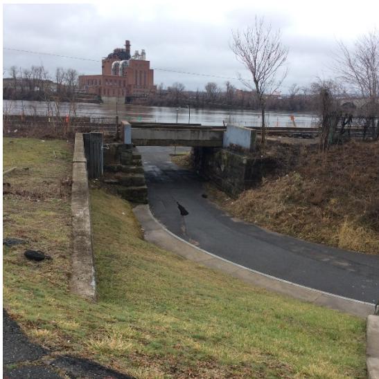
Figure 2-84: Unsafe Connection to Connecticut Riverwalk and Bikeway
