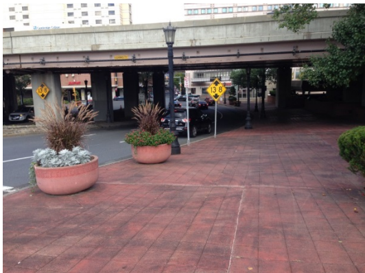
Figure 2-35: Boland Way Underpass
