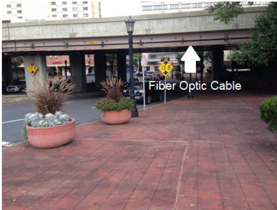
Figure 2-19: Fiber Optic Cable Attachment on I-91
