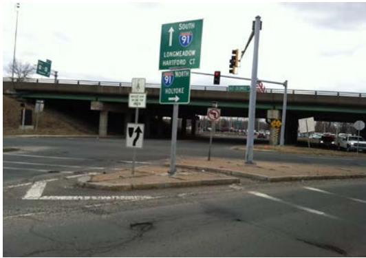
Figure 2-31: Main Street Underpass
