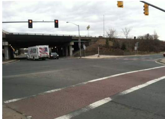
Figure 2-32: Broad Street Underpass
