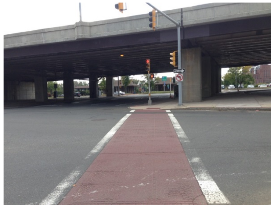
Figure 2-34: State Street Underpass
