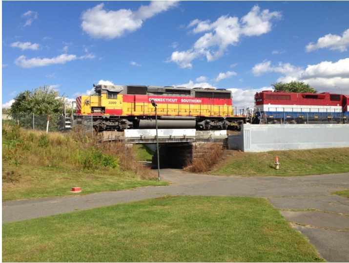
Figure 2-38: Underpass Below Tracks Off West Columbus Avenue
