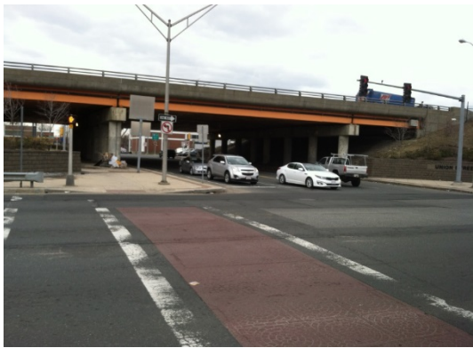
Figure 2-33: Union Street Underpass
