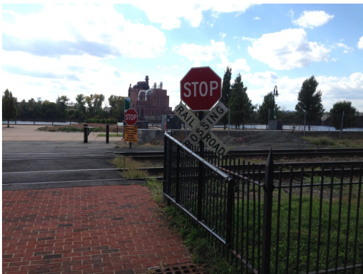
Figure 2-39: Passive At-Grade Highway-Rail Crossing at Riverfront Park
