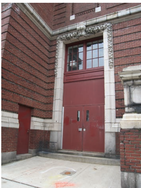
Many doors that were once important campus entrances are now locked egress doors, further confusing public access
