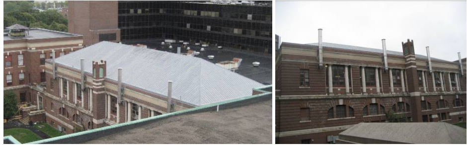
L- Viewed from South Building roof, with Tower in the background. R- Viewed from Collins Building; note the four exhaust stacks.
