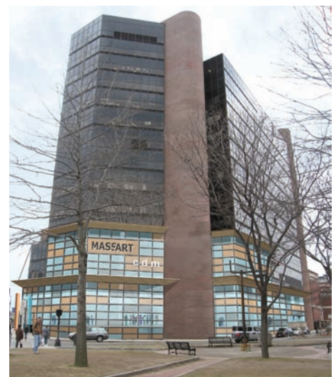
The new CDM at the base of the Tower
