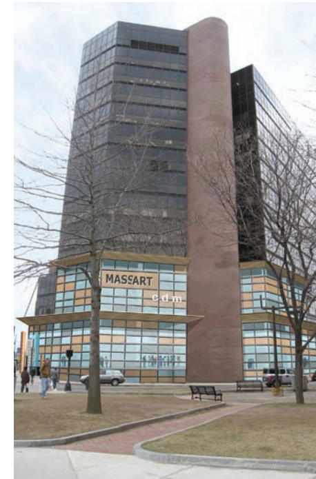
Stage 1 of MassArt's new Center for Design and Media* will have a prominent face on the Avenue of the Arts, with a portion of the Center occupying the unused space of the Tower portico and lending the building a fresh, new aesthetic
