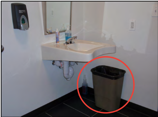
LOCATION | Student Counselling Offices Toilet Room
