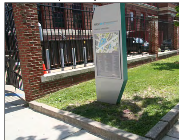
EXTERIOR - Palace/Tetlow curb and grass makes directory inaccessible
