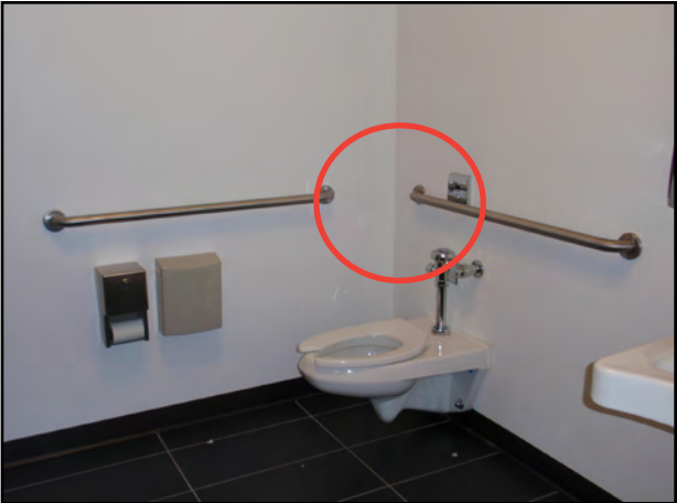
LOCATION | Student Counselling Offices Toilet Room
