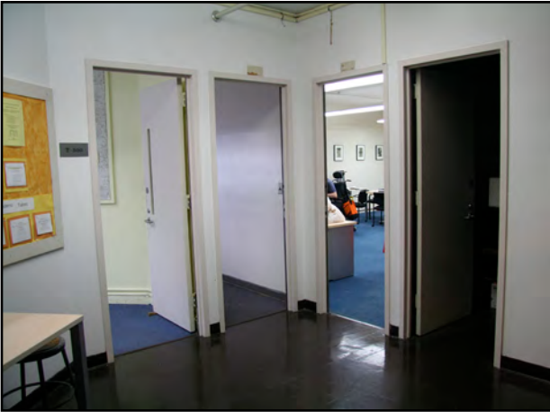
LOCATION | (T538 6" latch pull side clearance for corner door Learning Center)
