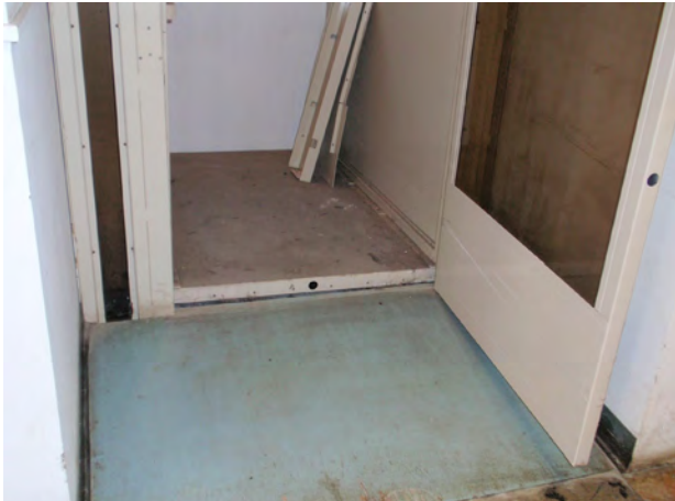
LOCATION | B10/208 Lift
