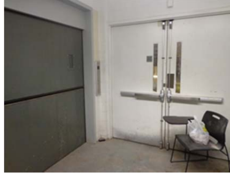
Figure 3.3.4 Freight elevator and Stair 1.
