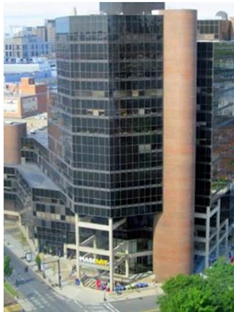
Figure 1 MCAD Tower Building
