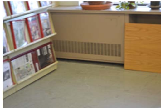
Figure 2.7.7 Exhaust fan at perimeter
