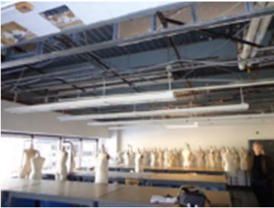
Figure 2.4.20 Inconsistent fireproofing
