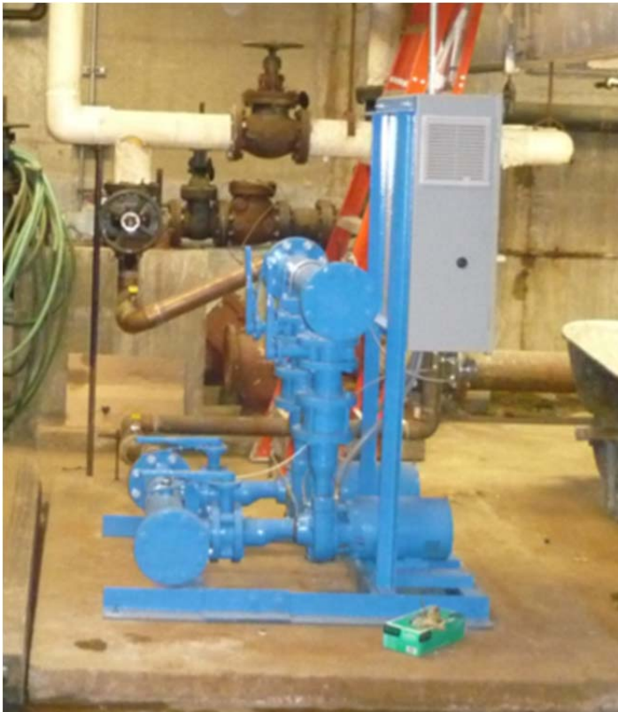
Figure 2.9.1. Duplex booster pump
