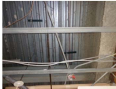
Figure 2.4.21 Inconsistent fireproofing
