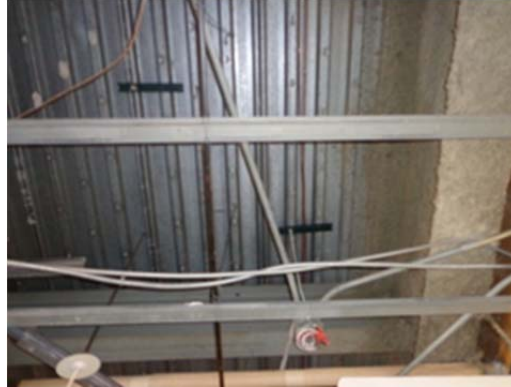
Figure 3.3.12 Inconsistent fireproofing
