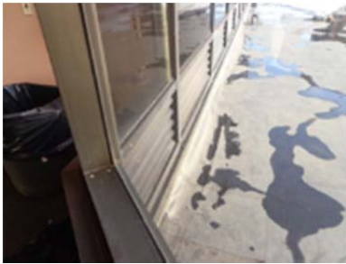
Figure 2.4.7 Water ponding
