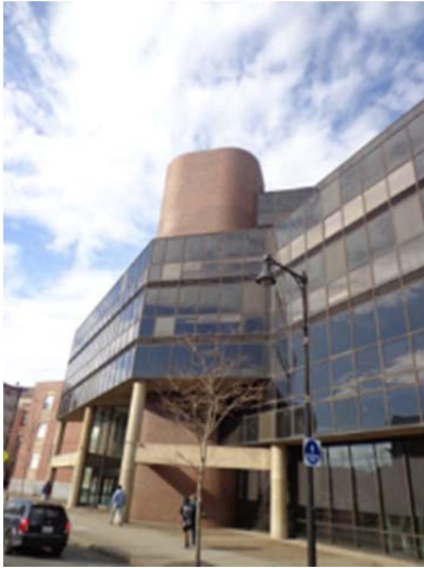
Figure 2.4.1 Concrete frame at street
