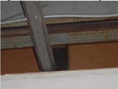
Figure 2.4.23 Inconsistent fireproofing
