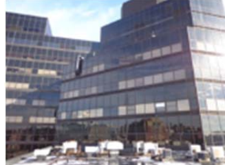
Figure 2.4.3 Curtain wall
