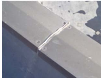
Figure 2.4.12 Exposed fasteners
