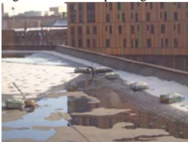
Figure 2.4.9 Sandbags on membrane
