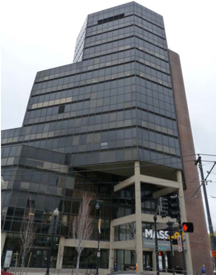
Figure 2.5.1 General Elevation of the Tower prior to the snap cap fastening
