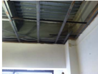
Figure 2.4.22 Inconsistent fireproofing
