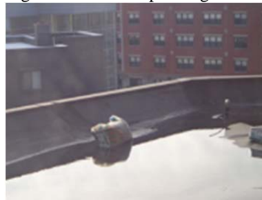
Figure 2.4.10 Sandbags on membrane
