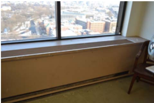
Figure 2.7.6 Unit ventilator
