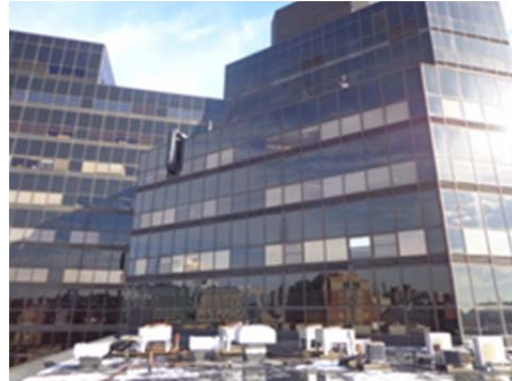
Figure 3.4.2 Tower curtainwall. Vision glazing is blocked up and/or blinds are drawn
