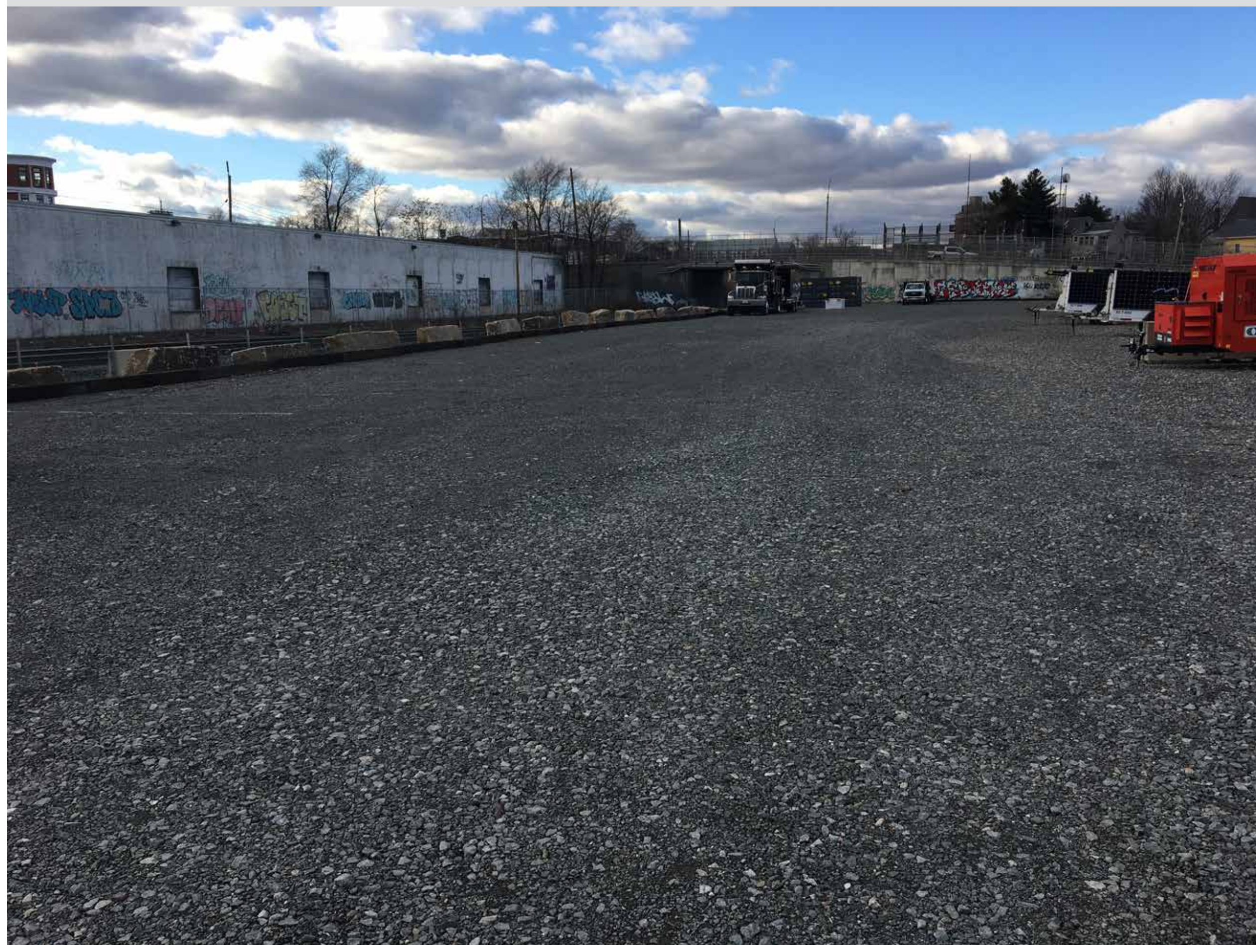
STATION AREA LOOKING WEST
