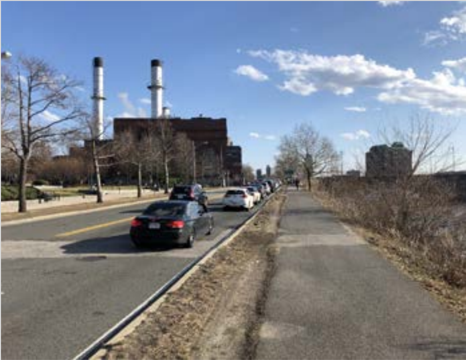
Existing conditions nearing the Western Avenue and Memorial Drive intersection
