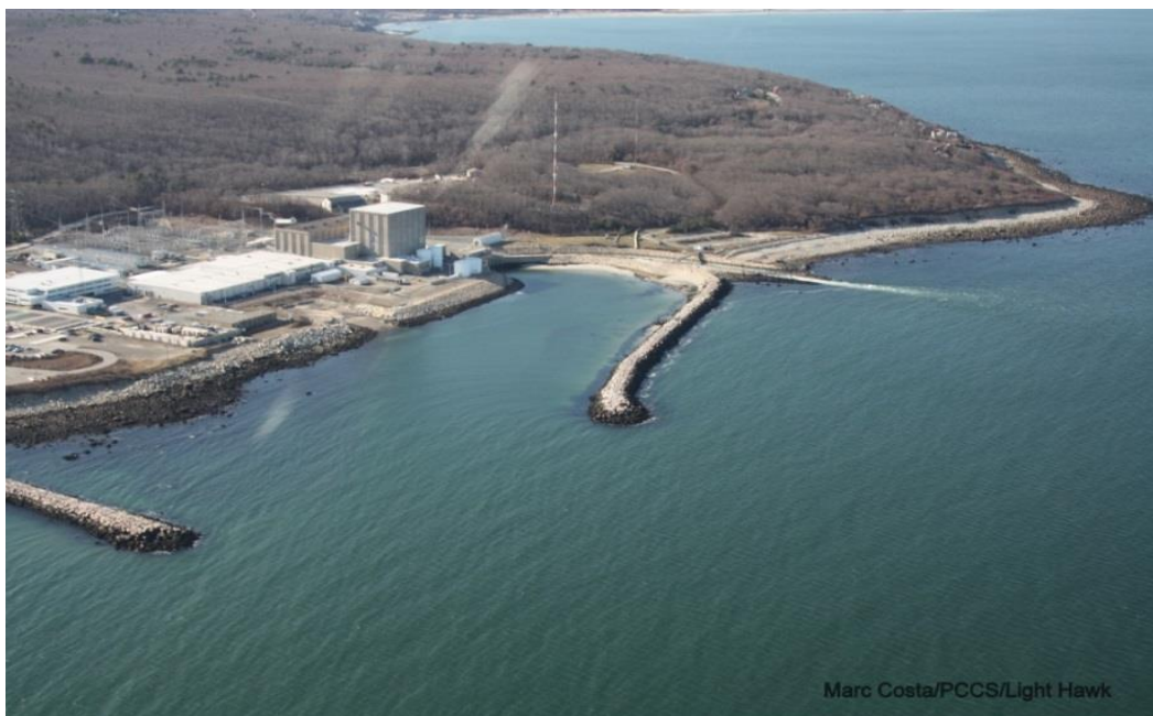
Figure 2. Pilgrim Nuclear Power Station, showing jetties, cooling water intake canal (center), and discharge channel (right). (Photo: Marc Costa/CCS/Light Hawk)
