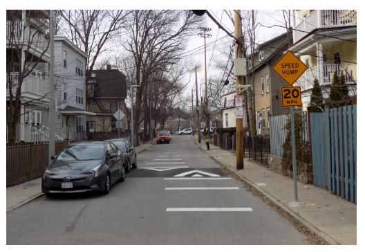
Bike boulevards are characterized by the use of traffic calming measures to reinforce 20 mph or lower operating speeds.
