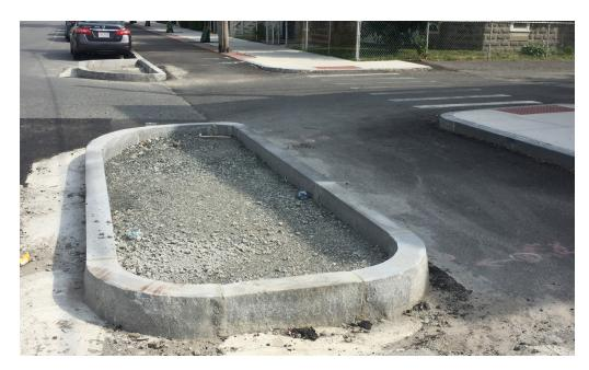
Incorporating protected intersection design principles does not always require the intersection of two separated bike lanes. For example, these under-construction corner islands where a separated bike lane intersects a side street will improve visibility for all modes and create crossing islands for people walking.
