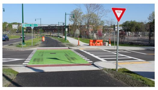
A two-way bike crossing under construction as part of the Casey Arborway project. This bike crossing features green colored pavement and is adjacent to a separate high-visibility pedestrian crossing.
