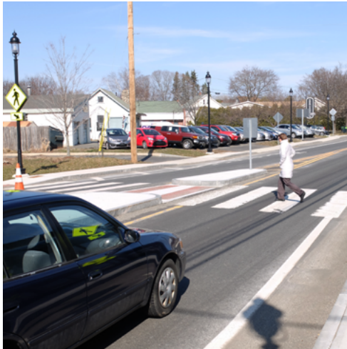
Figure 16. Pedestrian crossing islands improve pedestrian visibility and encourage yielding.
