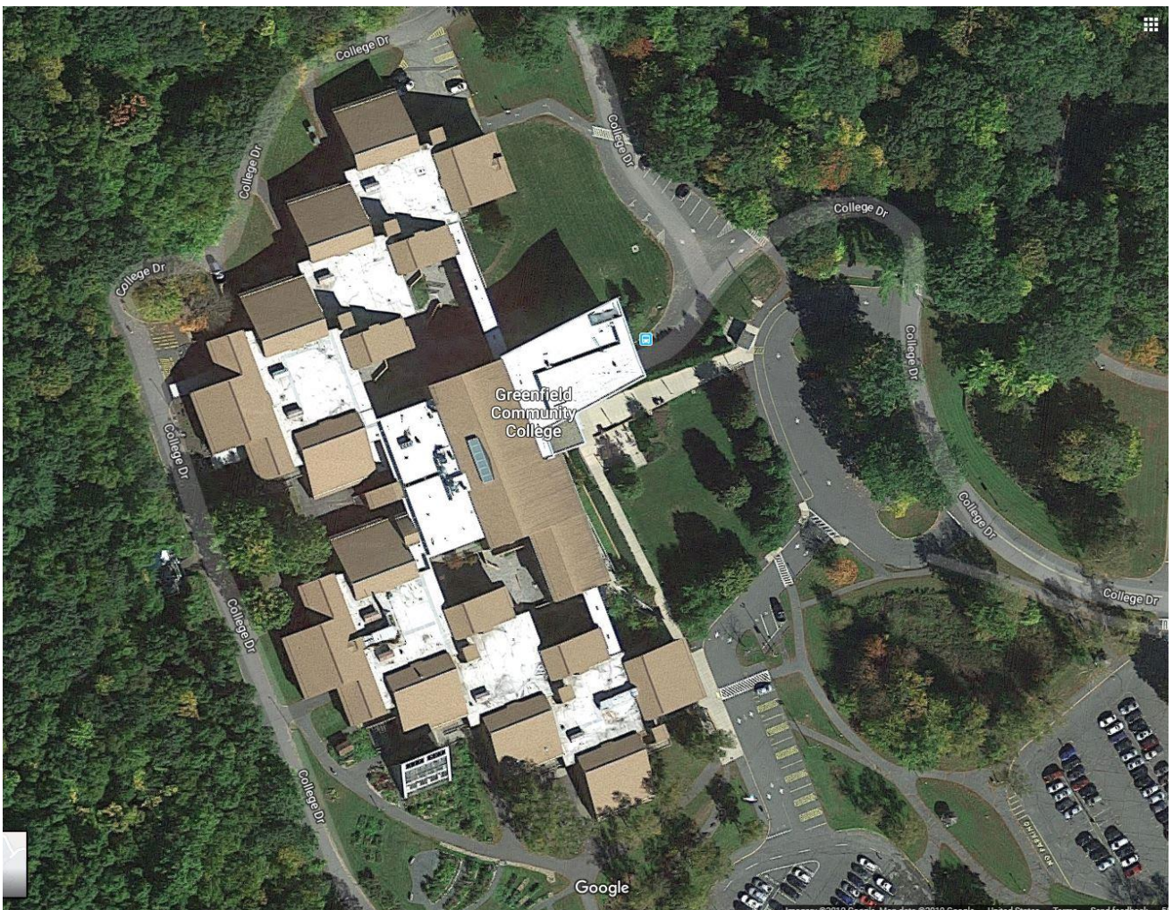
Greenfield Community College Main Building - View of Roof
