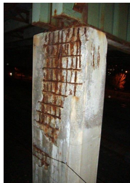
Deteriorated concrete column supporting the I-90 viaduct
