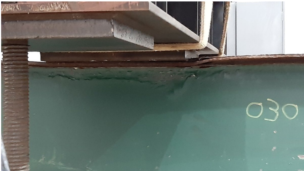
Figure 6.34: Web crippling observed underneath area of loading.
