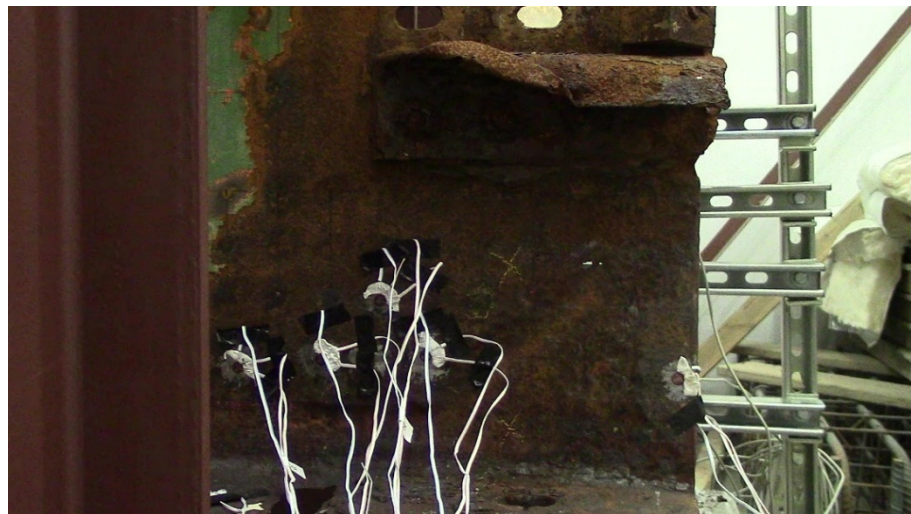
Figure 3.26: Instrumentation configuration at the end of Specimen 2.
