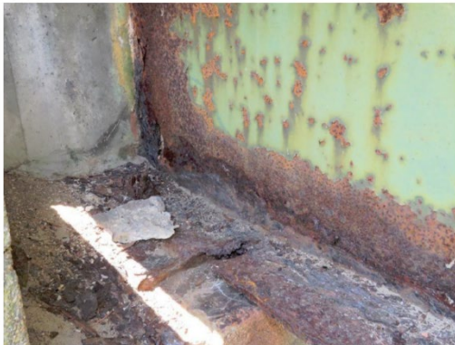
Photo 9: Beam #6 at the South end.
