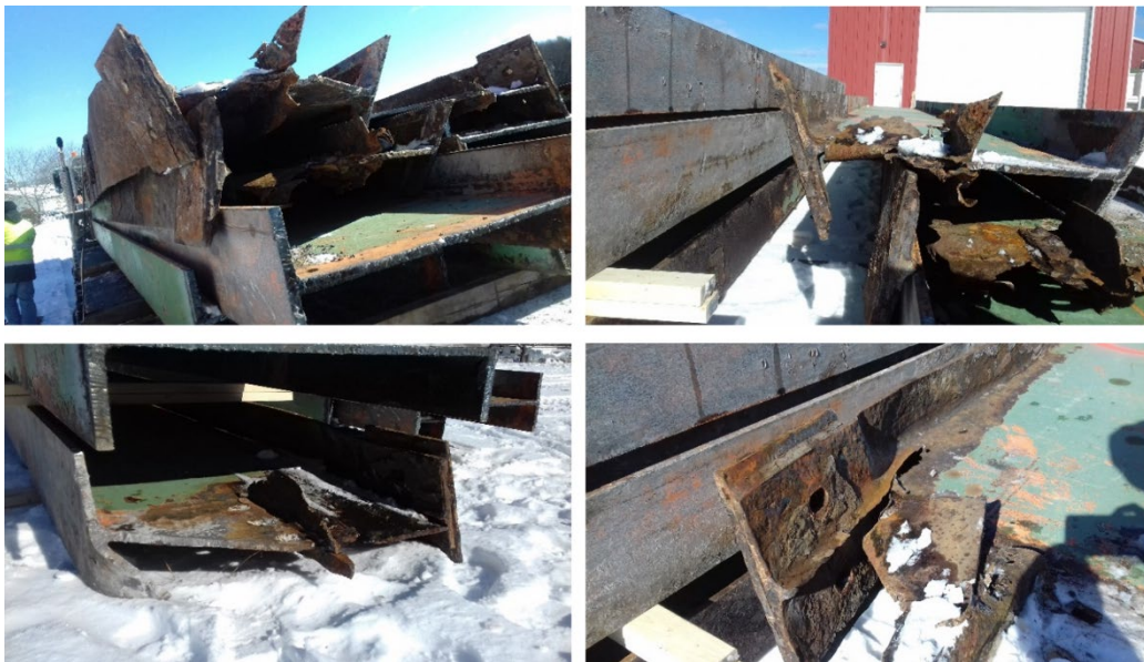
Figure 3.3: Distorted beams rejected for experimental testing due to condition.
