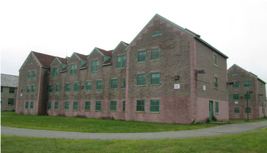
Photograph No. EX-7 Exterior of Main Housing.
