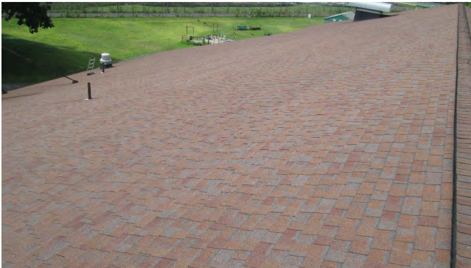
Photograph No. R-8 Shingle roof at Main Housing.
