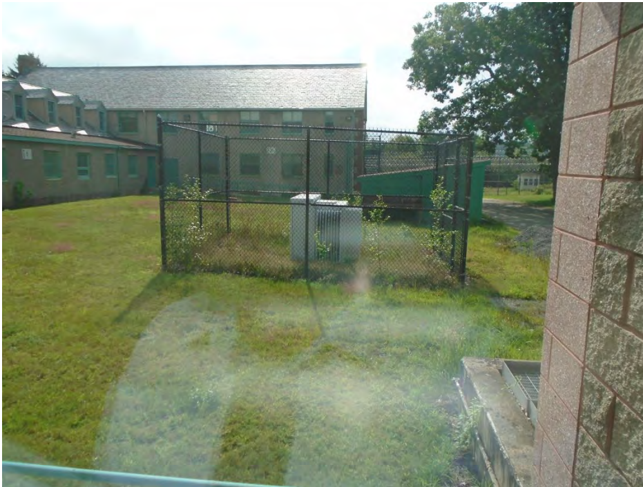
Photograph No. E-08
