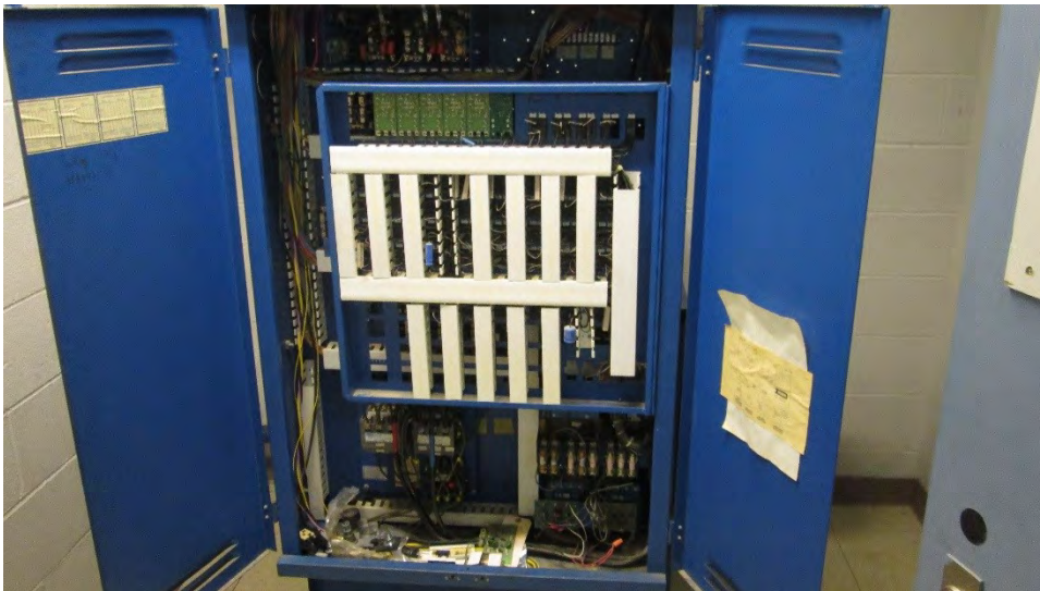
Photograph No. C-01
