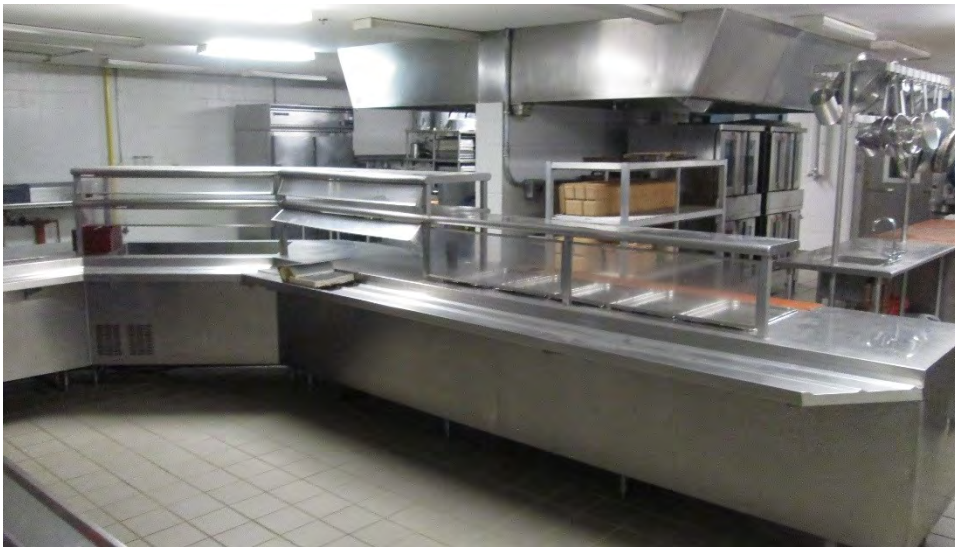
Photograph No. I-5 Kitchen.
