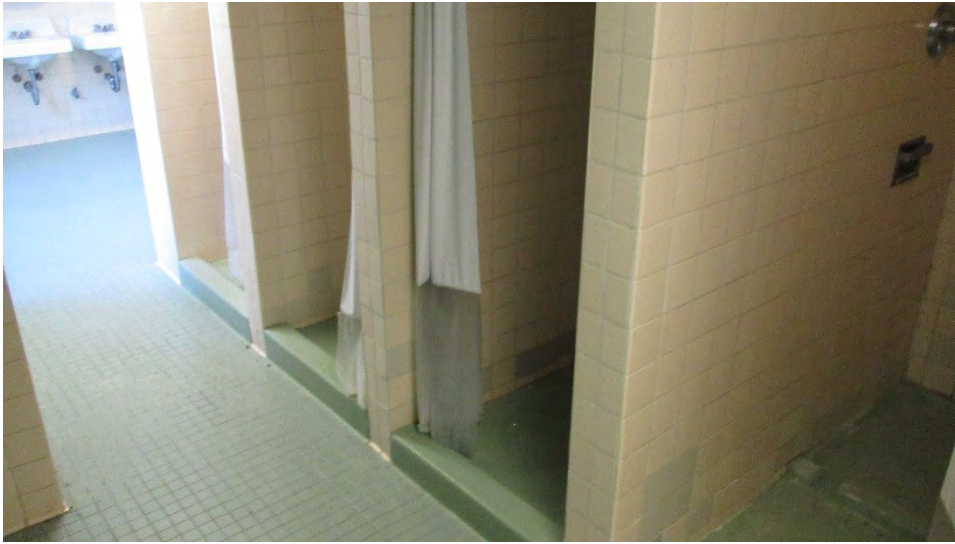
Photograph No. I-4 Showers at Main Housing.
