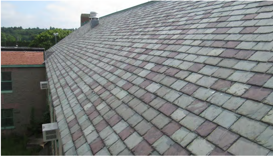
Photograph No. R-9 Slate roof at Administration Building.
