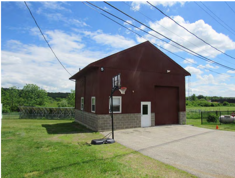
Photograph No. EX-10 Front Elevation of Automotive Garage
