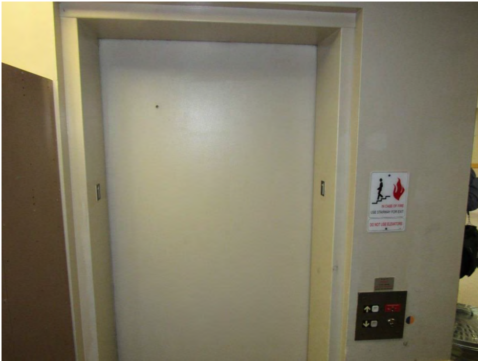
Photograph No. C-2 Elevator Hoistway Door
