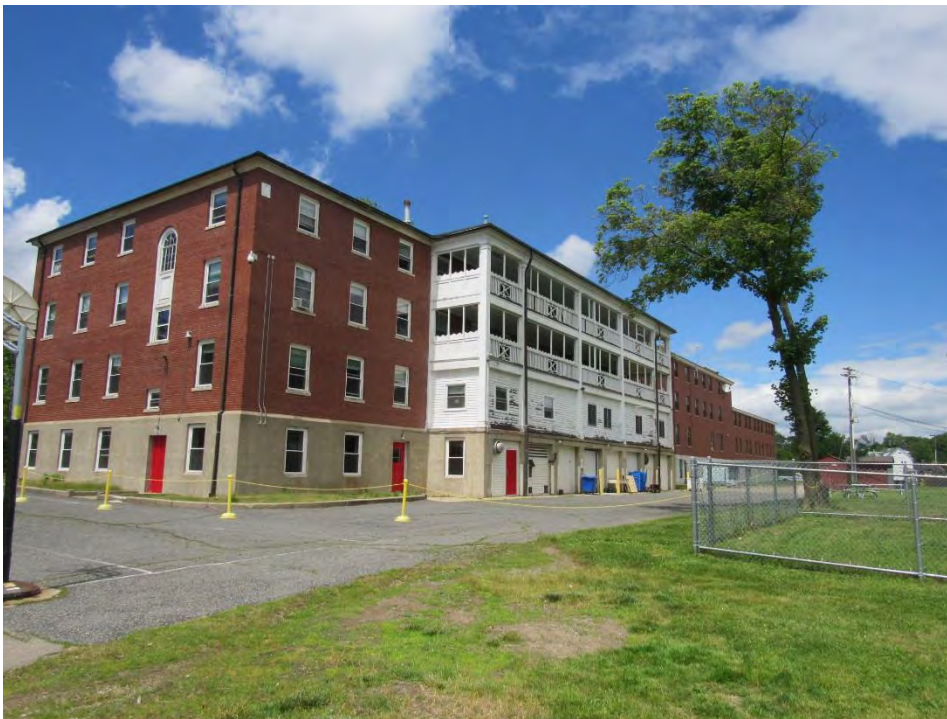
Photograph No. EX-8 Rear Elevation of Main Building
