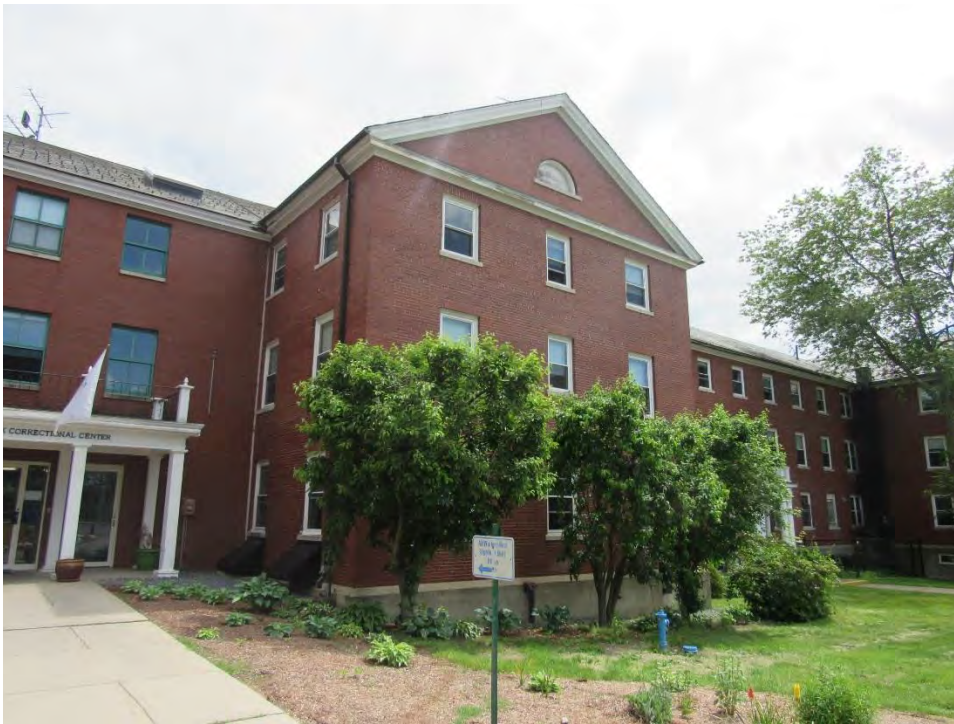
Photograph No. EX-4 Front Elevation of Main Building
