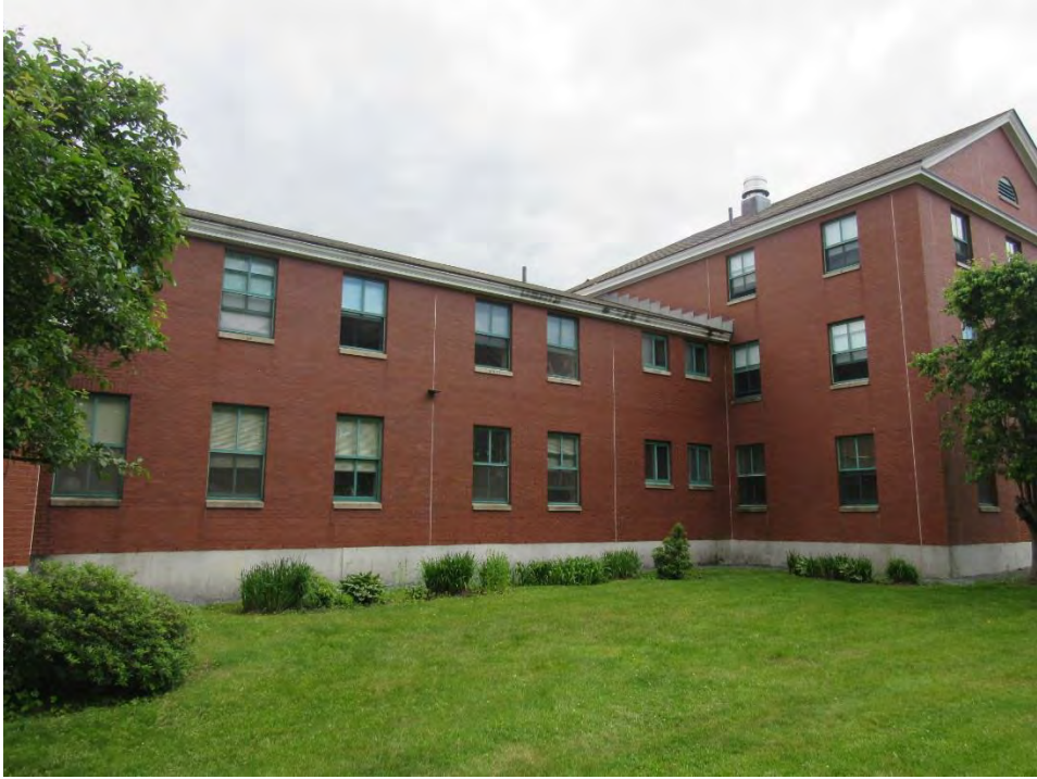
Photograph No. EX-3 Front Elevation of Main Building
