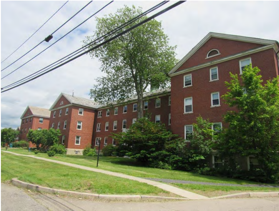
Photograph No. EX-7 Front Elevation of Main Building
