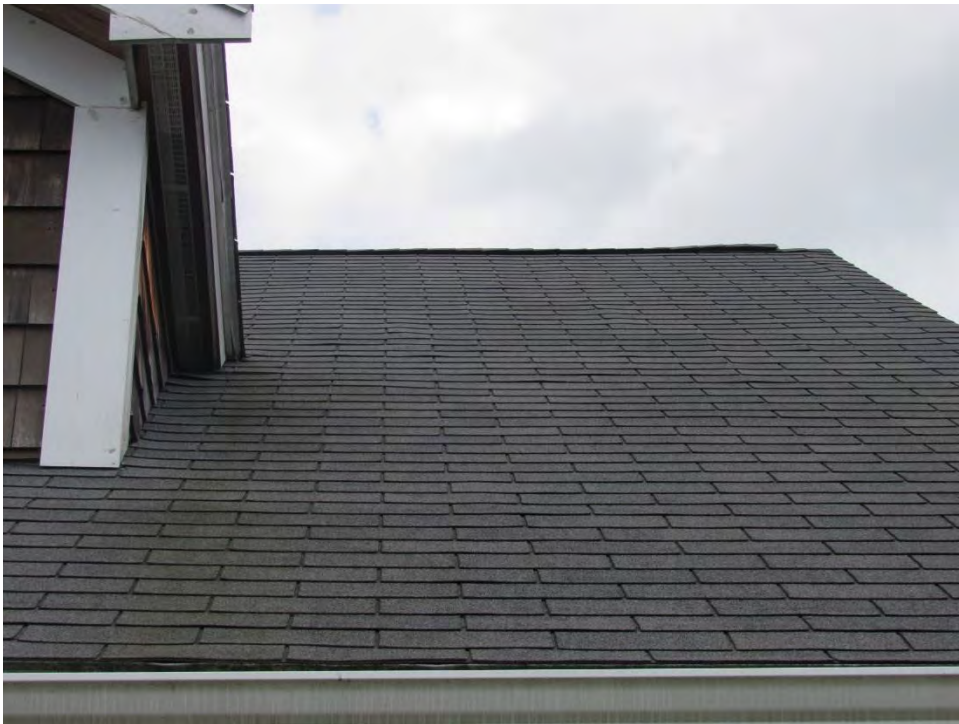
Photograph No. R-8 Shingle Roof at Reunification House
