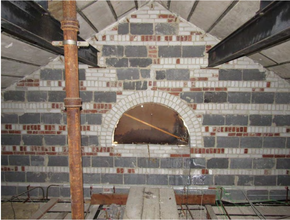
Photograph No. S-01 Roof Framing and Wall Back-Up at Main Building
