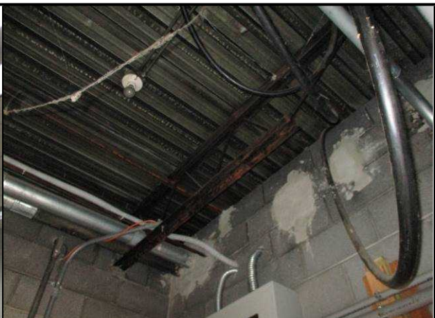
Corrugated metal roof decking and open-web steel joist.
