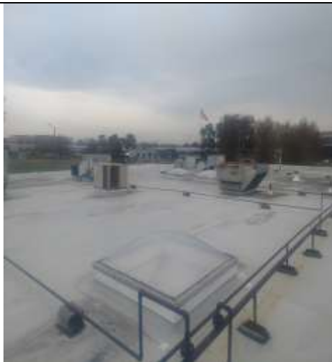
View of roof
