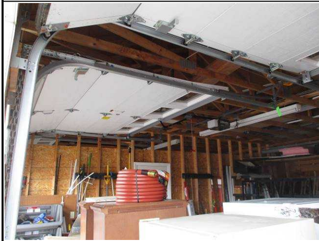
Maintenance garage building overhead doors.
