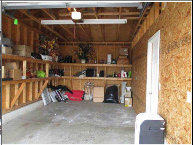
Maintenance garage building interiors.
