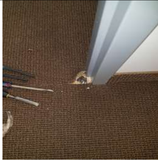
North office area floor tile beneath carpet
