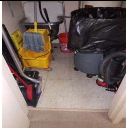
Janitor closet 2071, asbestos floor tile/mastic
