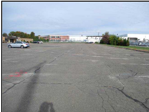
Asphalt-paved parking area at the rear of the Subject Building.
