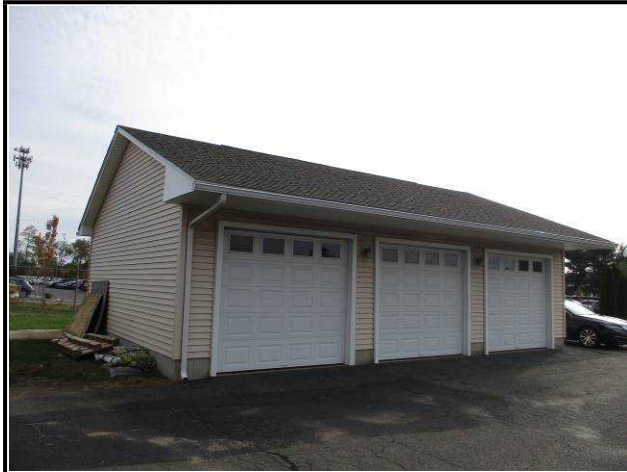
Maintenance garage building front and north side.
