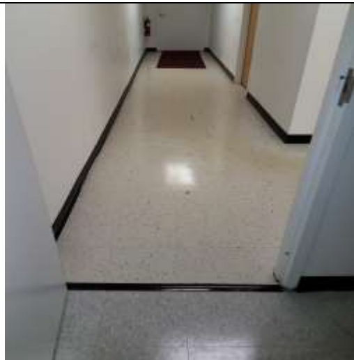
Kindred rear hall with double layer floor tile
