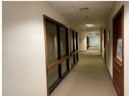
Typical interior construction.
