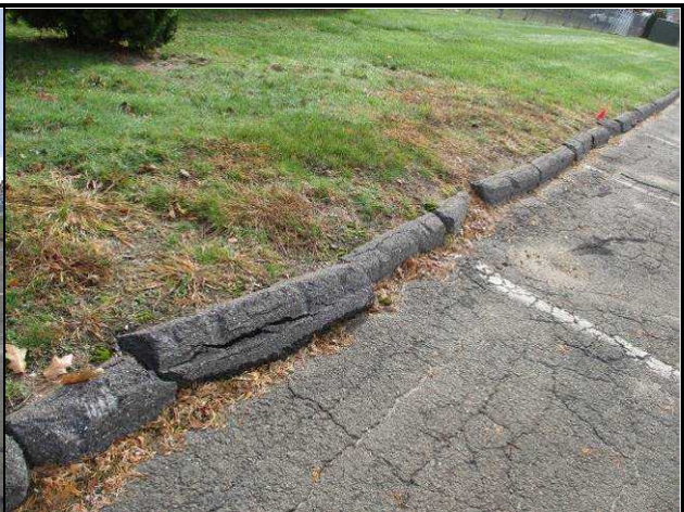
Extruded asphalt curbing at the rear parking lot.
