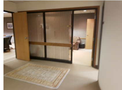
Typical interior glazed wall
