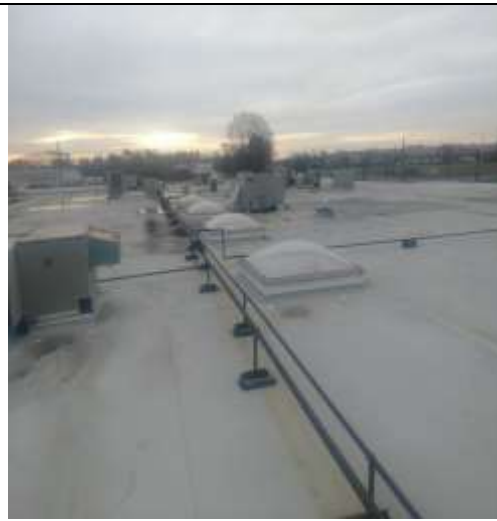
View of roof
