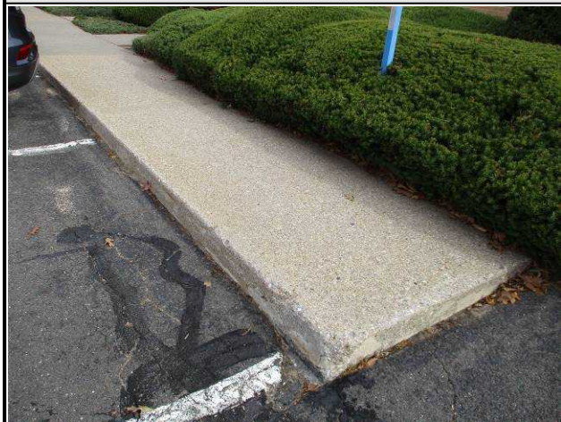
Typical concrete sidewalks.
