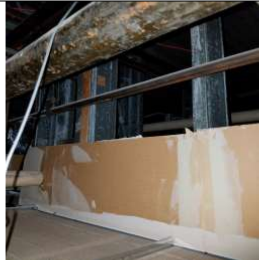
Old gypsum, tan JC and original wall stud
