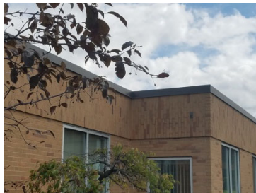
Brick veneer exterior with no parapet at roof.
