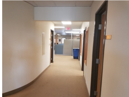
Typical carpet and hollow metal doorway
