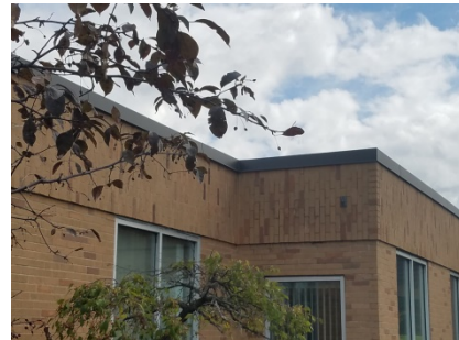
Roof is low sloping with no parapet.
