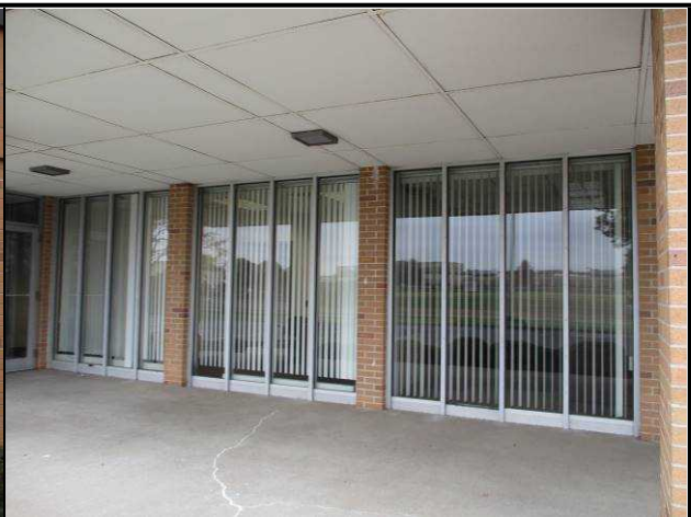
Typical storefront system at tenant entrances.
