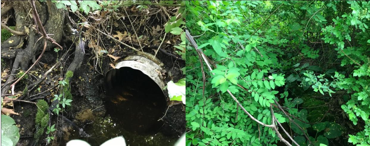
**Figure 23: The downstream corrugated metal pipe culvert at site S12.**
