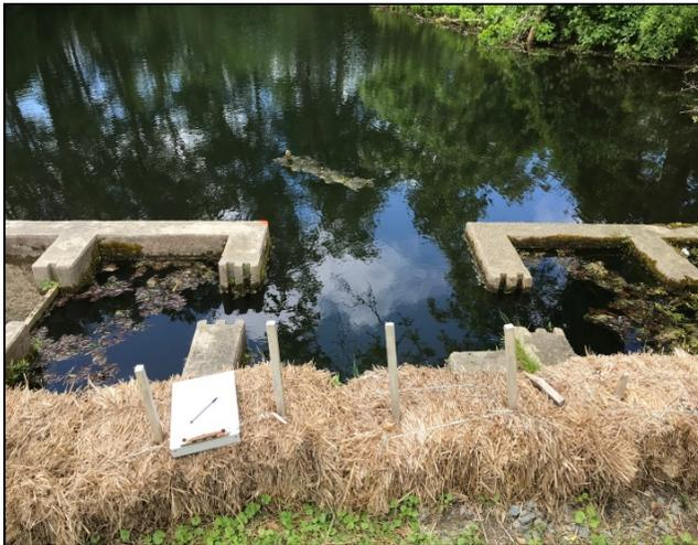
**Figure 3: Concrete dam/spillway structures controlling water levels on the upstream side of site S4.**
