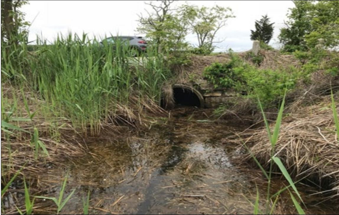
Figure 28: The culvert on the upstream side of site B1 is also covered with wrack, likely a result of high tides and storm surge from the blizzard in January 2018 and two northeasters in March 2018.
