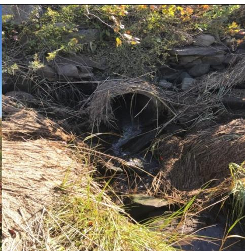
**Figure 64:** The downstream culvert was covered in wrack and is perched above a cascade caused by rip rap placed directly beneath the structure and continuing for some distance downstream at site Y3.
