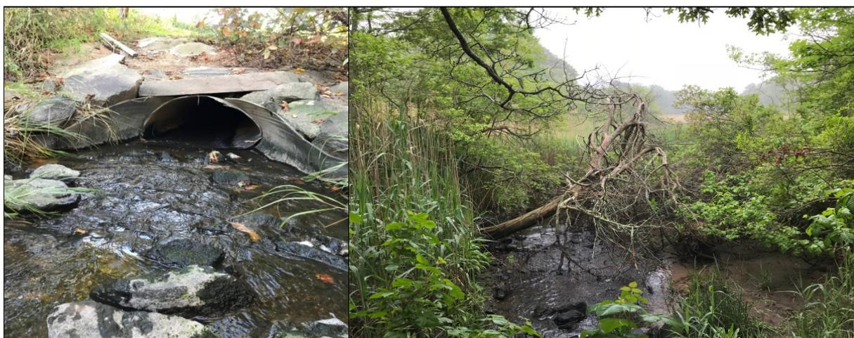
**Figure 48:** The metal culvert is partially collapsed on both sides of site B26. Shown here is the upstream side of the pipe, which is more profoundly collapsed than the downstream side.
