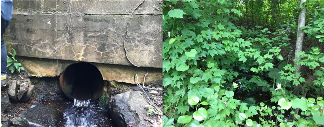
**Figure 34:** The downstream structure of site B3 is a small metal culvert that is slightly perched during typical low flow conditions.
