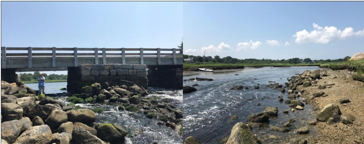
**Figure 54:** A stone support splits the bridge opening into two passageways for water flow and the bridge is heavily armored with large rocks on both sides at site Y1.
