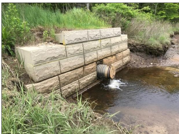
Figure 12: The flap gate on the downstream side of site S5 presents a tidal restriction, shown here at low tide.
