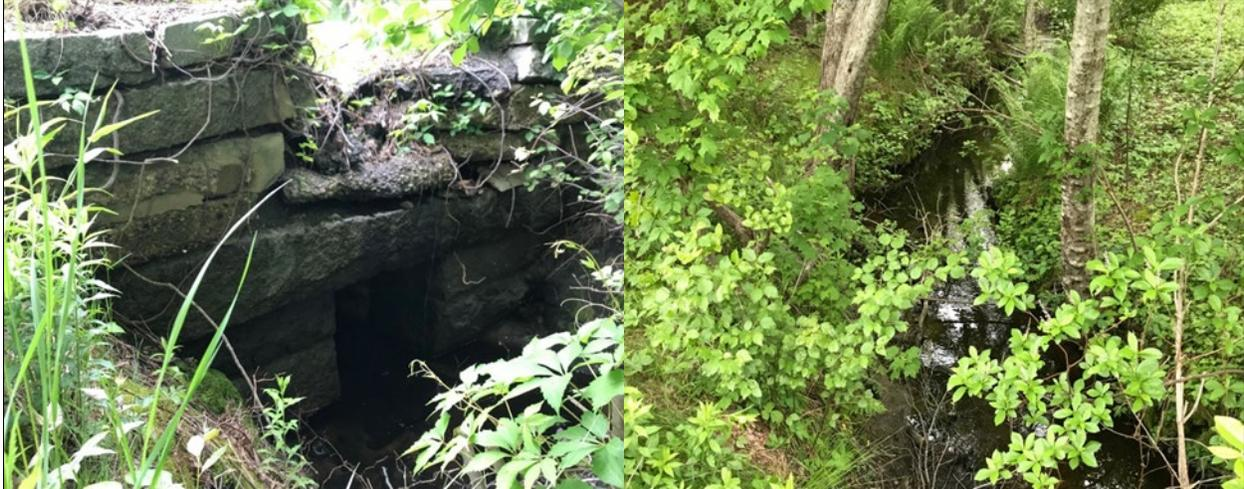
**Figure 31: The downstream box culvert at site B2 does not have a stone bottom, but does contain an artificial bottom that is not connected to the structure. Notice the erosion occurring directly above the culvert opening from road runoff.**
