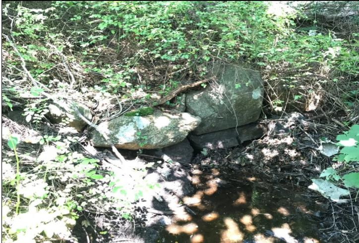
**Figure 69:** Field observers were unable to identify what kind of structure was covered by the stone at site Y4, shown here on the upstream side. Due to the small opening beneath the stone, debris has accumulated at the crossing.
