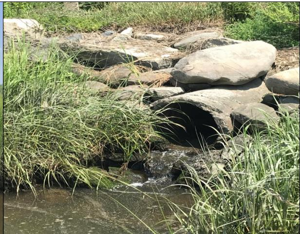
**Figure 60: The downstream structure is armored with stone and is perched above the creek at low tide at site Y2.**
