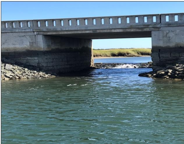
**Figure 45: View of the bridge from the downstream marina. Notice the perch created by the rip rap located on the upstream side of site B25.**
