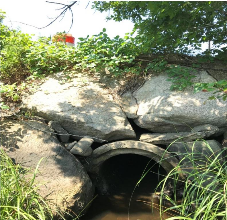
Figure 66: The upstream culvert has stone placed around the opening, and is beginning to deteriorate, especially the lower half of the structure at site Y3.
