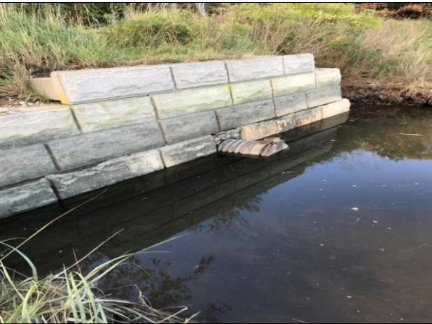
**Figure 15: The downstream flap gate at site S5 shown at high tide.**
