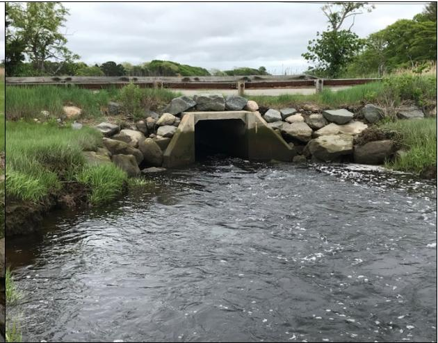
**Figure 21:** The downstream box culvert with wingwalls at site S10. Stone has been placed around both the upstream and downstream structures to help armor the crossing and minimize erosion.
