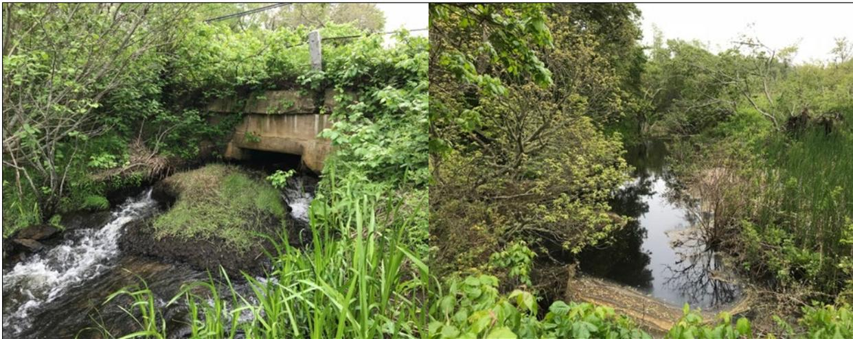
**Figure 37: A large mass of peat is partially blocking flow on the downstream side of site B7, most likely rafted up during the blizzard in January 2018 or the northeasters in March 2018.**
