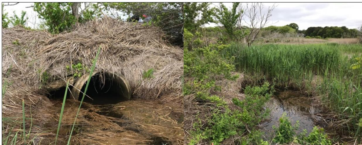
**Figure 26: The downstream culvert is covered in wrack, indicative of how the structure was impacted by the blizzard in January 2018 and northeasters in March 2018 at site B1.**
