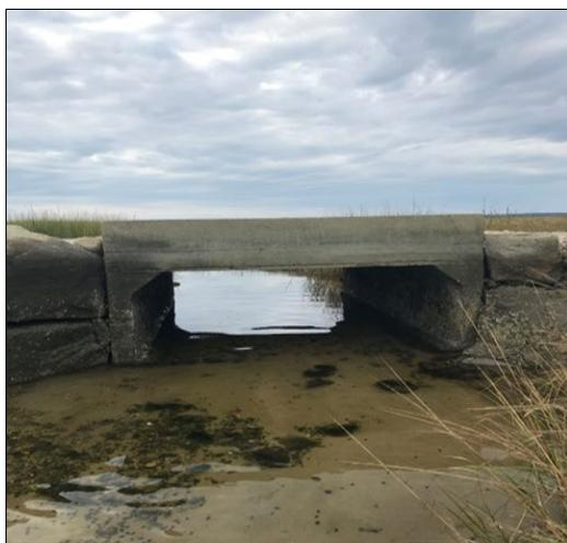
**Figure 41: The upstream side of site B23. The structure is in good condition and rock retaining walls have been put in place around the opening to limit erosion and washout of the trail.**
