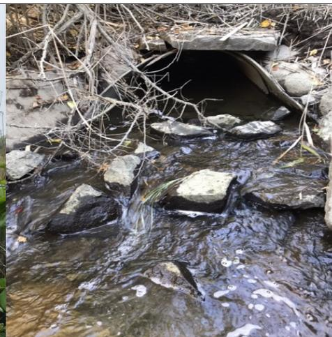
**Figure 51: The downstream creek has an area of rip rap that is creating a cascade from the culvert and resulting in increased water flow velocity at site B26.**
