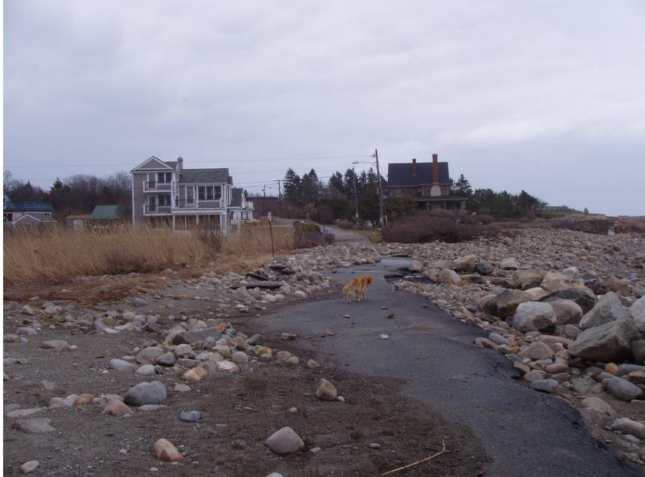
Photograph 4.5. Damaged pavement and overwashed sediment after a recent storm on a barrier beach. Photograph courtesy of Eric Hutchins, National Marine Fisheries Service.
