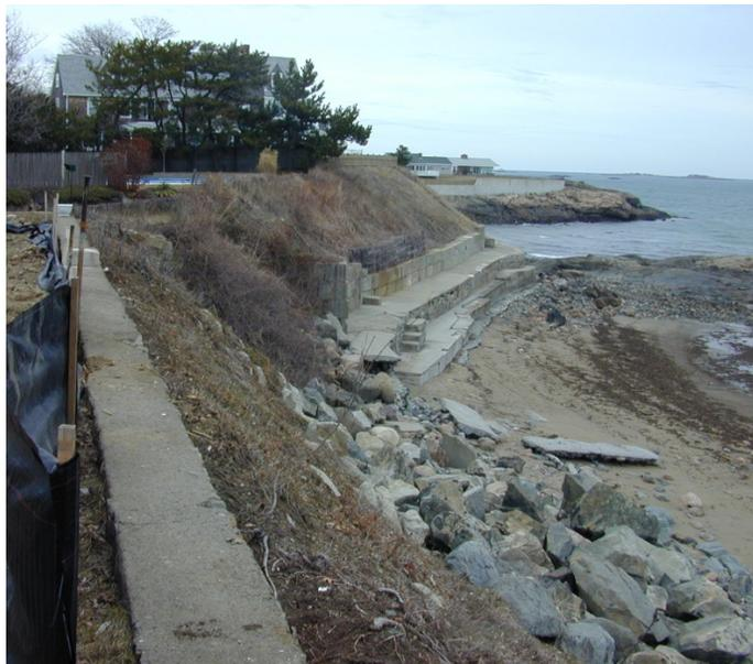
Photograph 4.6. Pre-existing riprap on coastal bank and coastal beach. The rocky intertidal shore can be seen in the distance.
