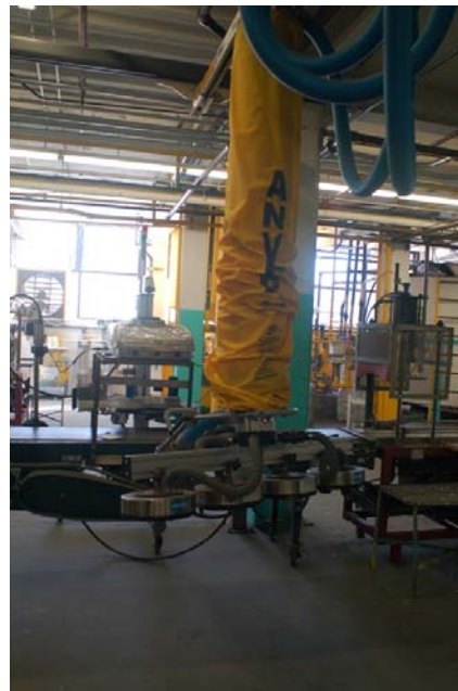
Recently installed overhead lift for moving paint pails that protects workers from back injuries.
