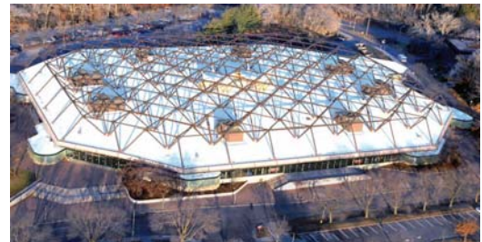
The 158,000-square-foot roofing system at the Carver-Hawkeye Arena at the University of Iowa features membrane Sika Sarnafil recycled from the old roof, which had been damaged by a severe storm.
