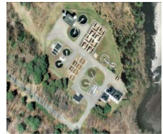
Marlborough's Wastewater Treatment Facility
