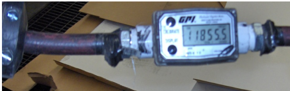
Flow meter installed by Massachusetts Container Corporation on hose used for equipment washing
