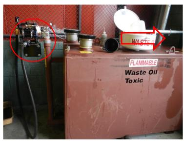
This waste oil management system works with waste oil collection caddies (left) that are wheeled from the vehicle to the shop's waste oil storage tank (right). The oil is emptied from the caddies into the
