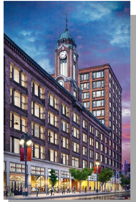
The Sibley Building. Image Credit: NYSERDA.
