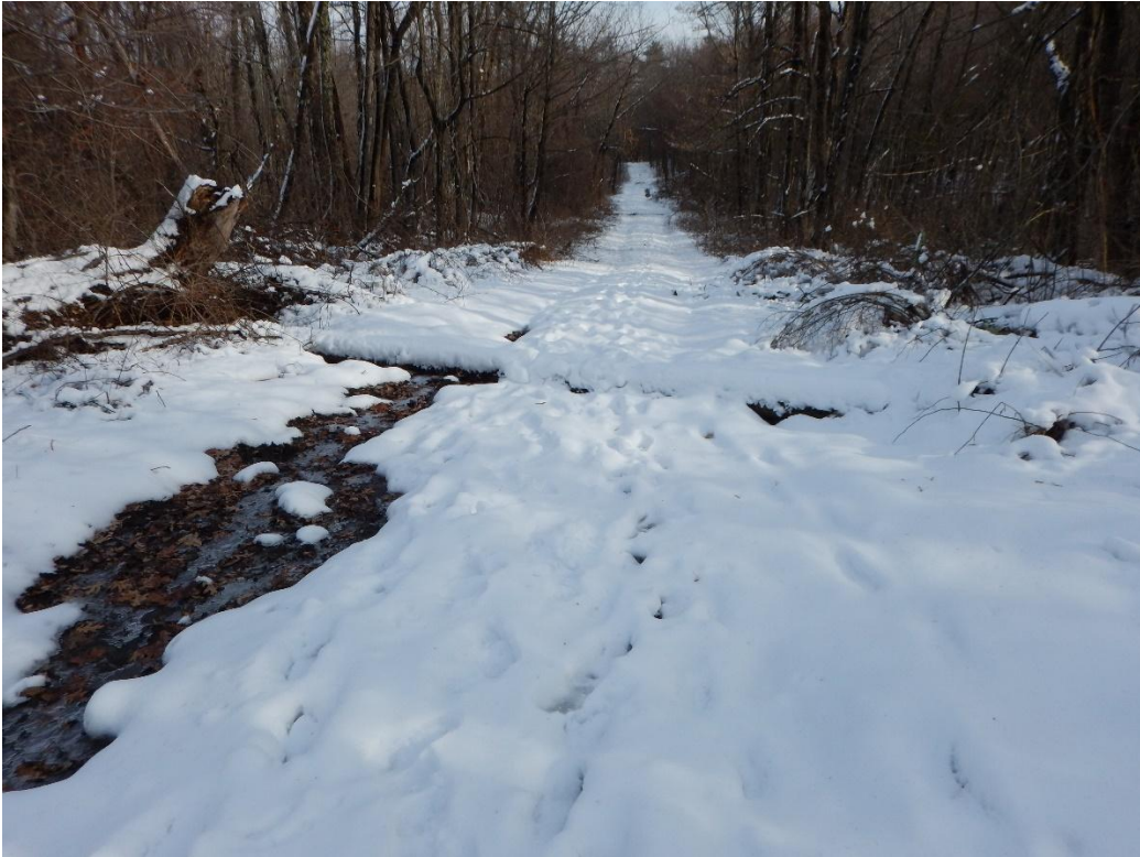
A. One of three water bars installed on the former Gill Road in order to prevent water from running down the road and causing erosion.
