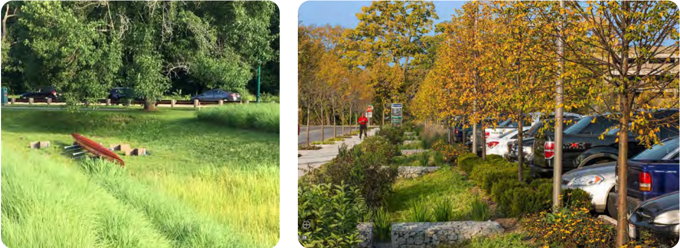
Figure 2-28. Examples of green infrastructure for treatment of parking stormwater runoff: Bioretention swales at Harry Parker Boathouse, Brighton, MA (left) and Christ Hospital, Cincinnati OH (right). Image credit (left): DCR, (right): www.OJB.com.
