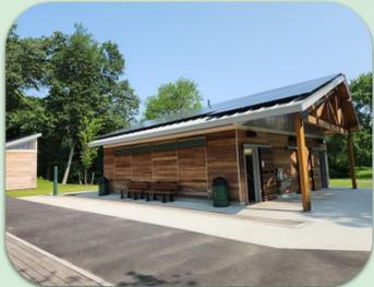
The Task Force supports net-zero goals in new construction projects. The Shannon Beach Bathhouse, completed in 2023, includes a 14kW solar array with a backup battery system to provide 100% of the facility's electricity needs.
