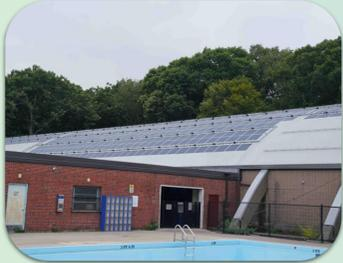
In 2022, the team identified an innovative thin-film solar PV technology that could be cost-effectively installed on barreled ice rink rooftops. Solar PV has been installed on two rinks, effectively eliminating grid electricity use. The team plans to deploy this technology on three additional sites over the next year.
