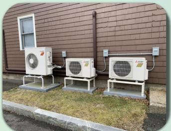
The Net Zero Task Force led a portfolio-wide analysis of fossil fuel-based heating equipment at DCR sites and developed a strategy to replace this equipment with air-source heat pumps as it reached the end of life. Air source heat pumps and water heater systems were installed in 41 buildings in FY23, with another 40 sites planned for FY24.
