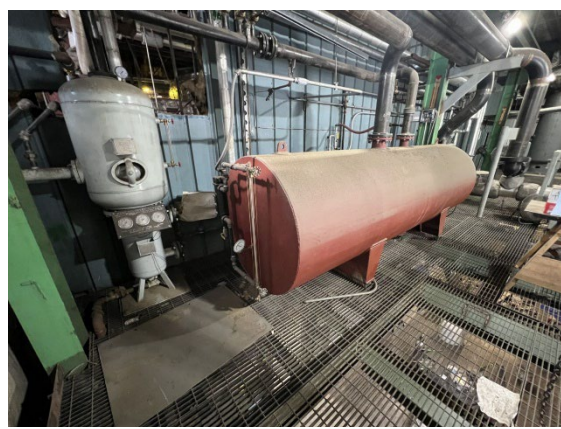
Flash tank with shell and tube heat exchanger (L) and condensate reservoir (R)
