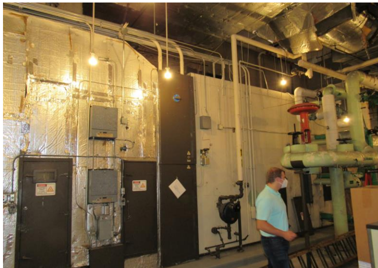
Photo 1 –Typical Air Handler and Return Fan
