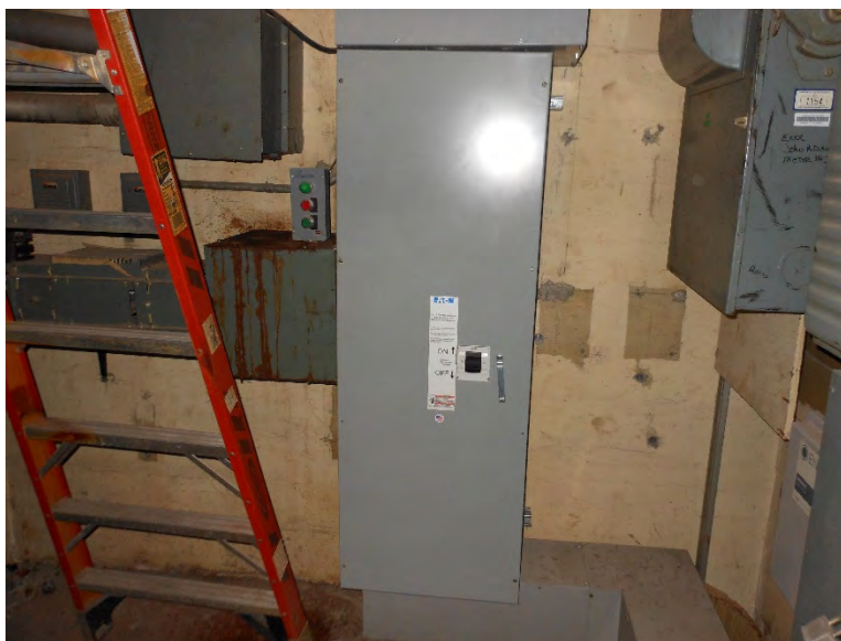
Picture 7 - Headquarters Building Main Electric Room 005 – 800A Switch
