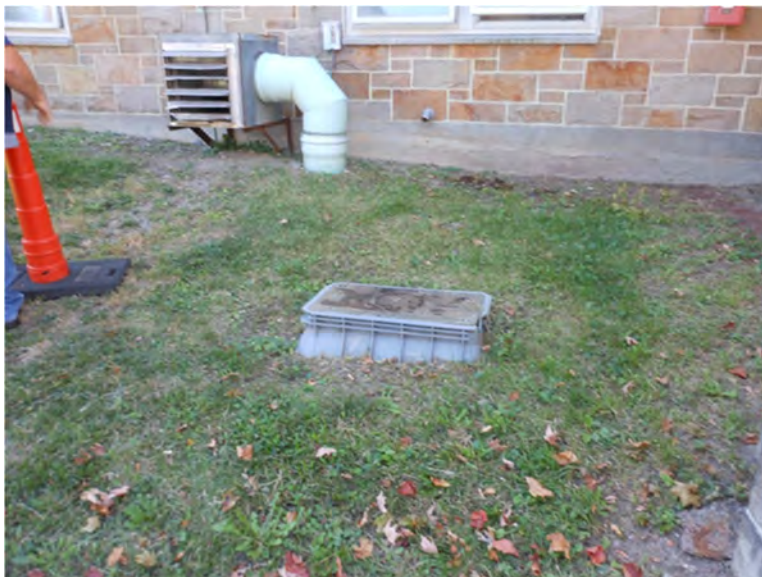
Picture 13 - Keville Building – Underground 208/120V Electrical Service Handhole
