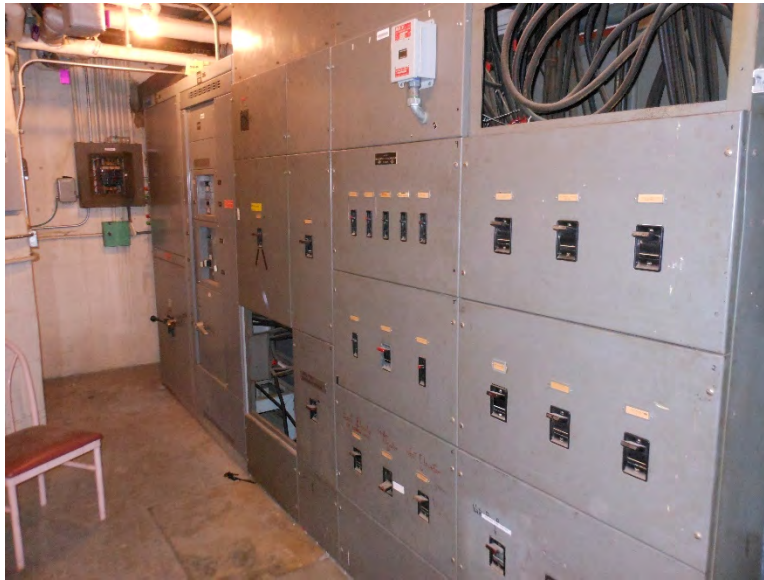
Picture 17 - Quigley Room B16 – 1600A, 208/120V Switchboard
