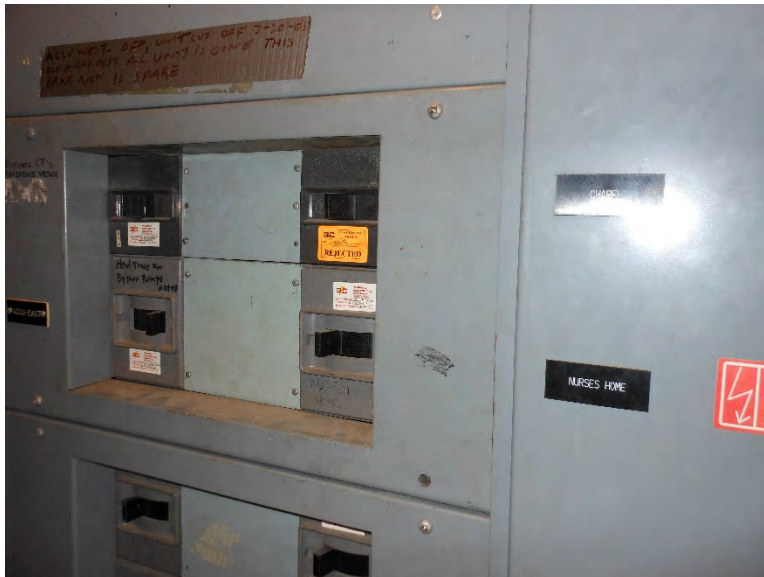
Picture 18 - Quigley Room B16 – 1600A, 208/120V Switchboard – Feeder to Chapel Panel
