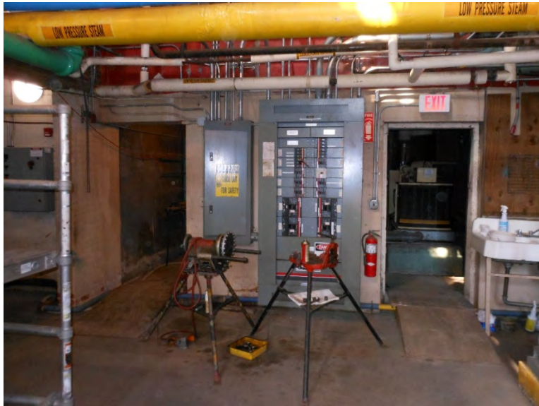
Picture 9 - Power Plant – 600A 208/120V Panel 'LP1'
