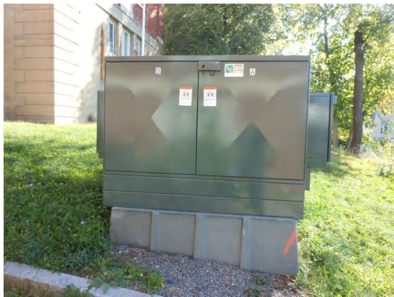
Picture 4 - Pad Mounted S&C Primary Switch
