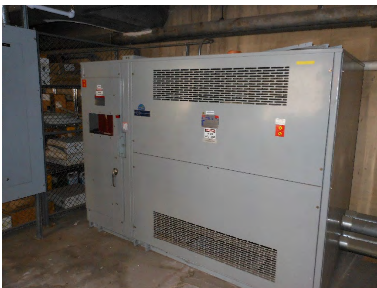
Picture 11 - Sullivan Building – 500kVA Unit Substation
