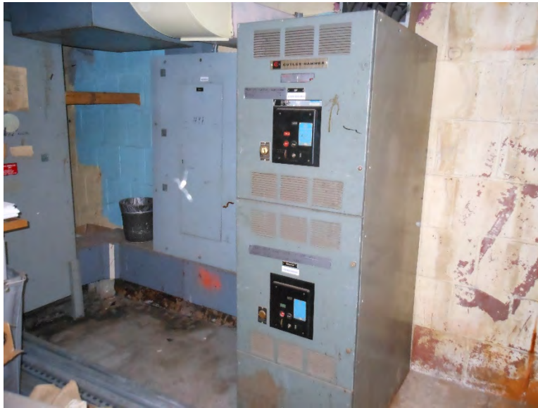
Picture 15 - Quigley Room B17 - 1600A, 208/120V Key Interlocked Manual Transfer Switch
