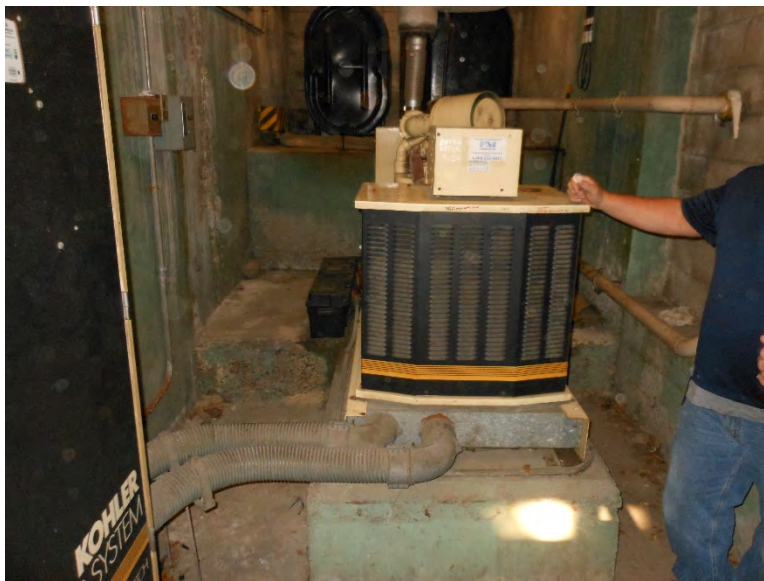
Picture 10 - Power Plant – Diesel Standby Generator & Automatic Transfer Switch
