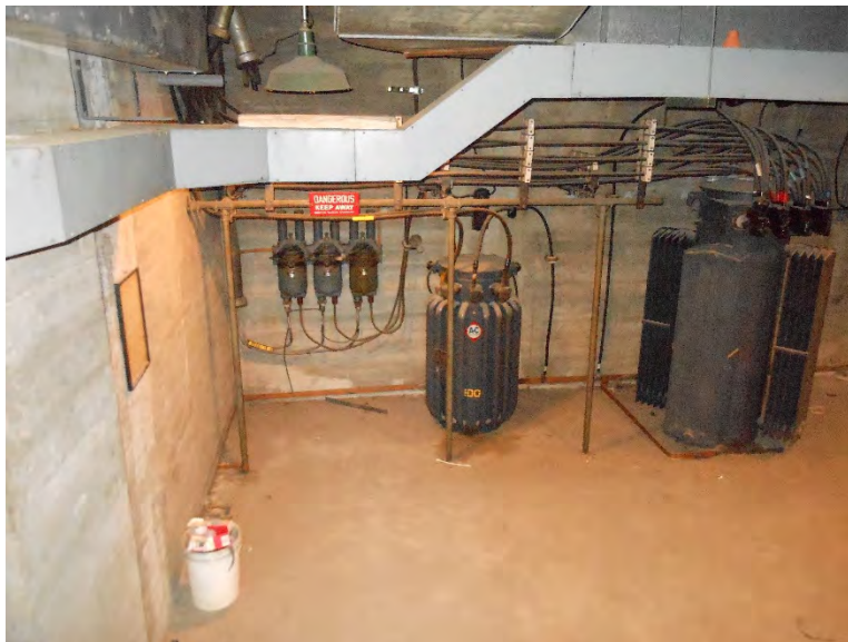
Picture 14 - Quigley Vault #2 -500kVA, 3-phase and 100kVA, single phase Transformers
