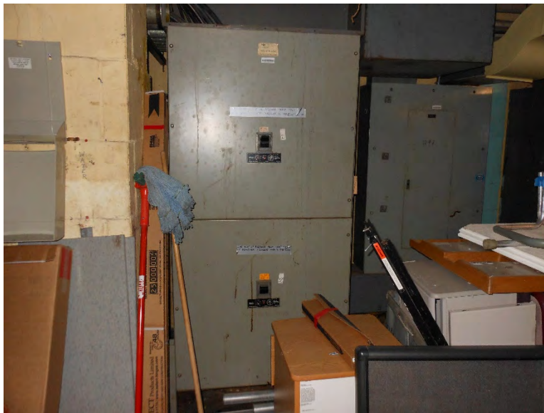
Picture 16 - Quigley Room B17 – 800A Circuit Breakers
