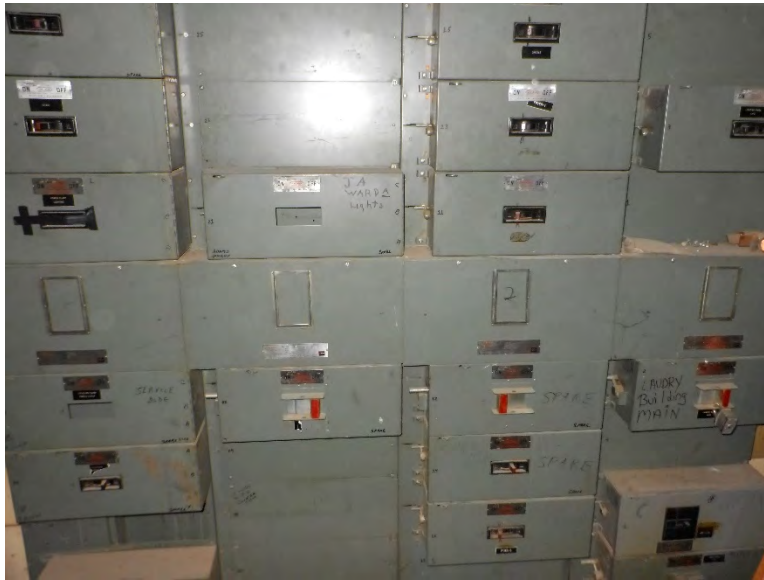
Picture 8 - Headquarters Building Main Electric Room 005 – 208/120V Switchboard
