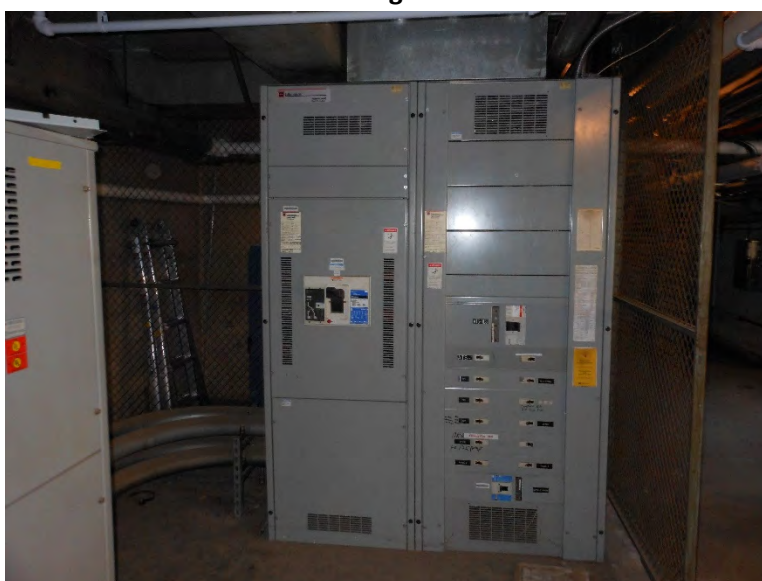
Picture 12 - Sullivan Building – 1600A, 208/120V Main Distribution Panel
