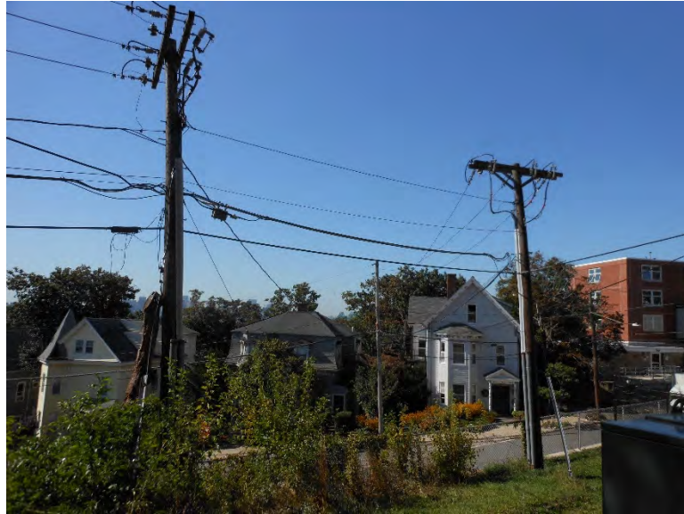
Picture 3 - Overhead 4160V Electrical Services (Line A and Line B)
