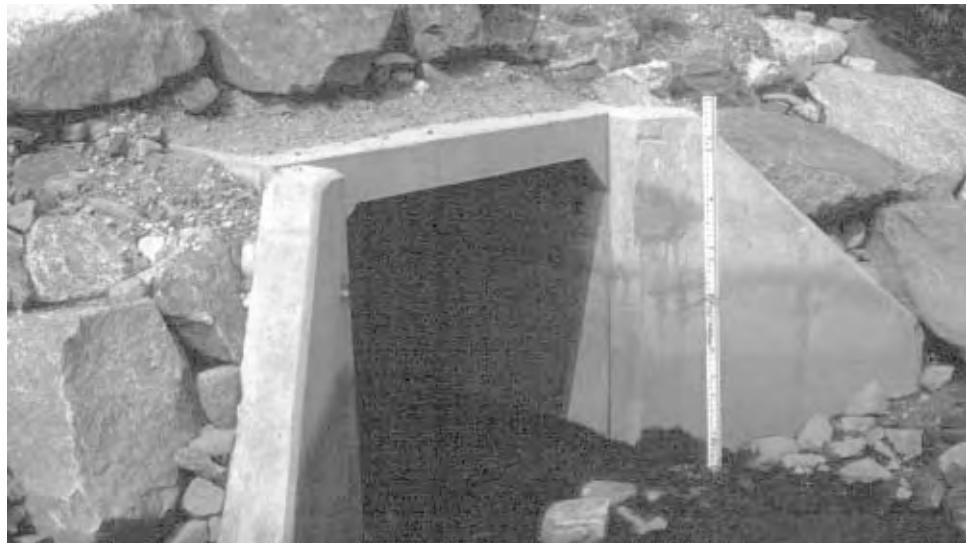
A staff gauge installed on a culvert. Photo: CZM Staff Photo
