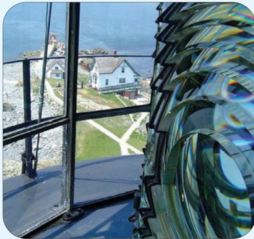
View of the Boston Harbor Lighthouse keeper's house on Little Brewster Island. Second order Fresnel Lens dates from 1859.
