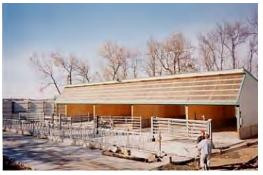
Figure 3. Open sided, single slope roof shed is one of the most common housing structures.
