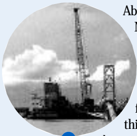
BARGE LAYING A NATURAL GAS PIPELINE
