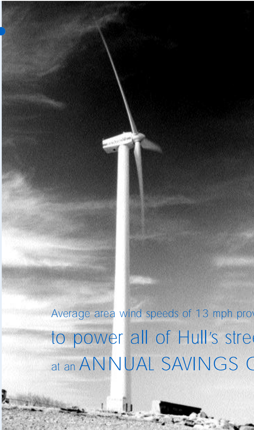
HULL MUNICIPAL LIGHT COMPANY'S WIND TURBINE ON POINT ALLERTON.
