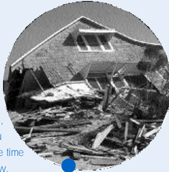
HURRICANE FRAN DOES SOME SERIOUS DAMAGE IN NORTH CAROLINA.
