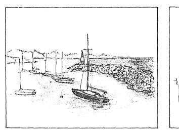
Jetties are linear barriers built of large rock or concrete. They are positioned to reduce the effects of storm wave surge or the force of strong currents. Jetties may be built parallel to offshore bays and river mouths to protect boat harbors or perpendicular to the shore to protect navigation channels of harbors and marinas.
