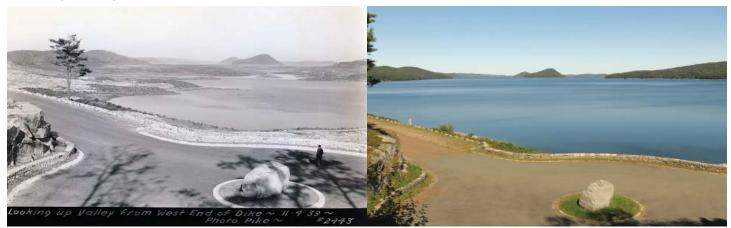
he flooding of the Swift River Valley to create the Quabbin Reservoir commenced on August 14, 1939 and took seven years before the reservoir reached capacity. Two massive impoundment structures hold back the 412 billion gallons of water of the reservoir: the Winsor Dam blocks the flow of the Swift River and the slightly smaller Goodnough Dike several miles to the east holds back water from the Beaver Brook drainage.
