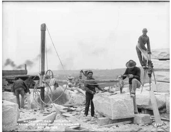
An example of one of the 8,800 detailed images of the Boston drinking water system's early construction now available through Digital Commonwealth.
