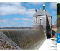
shed so that a major storm event, with the right combination of conditions, could produce enough inflow to overtop the dam. For that situation, based on a detailed analysis, MWRA constructed a parapet wall (also known as a wave wall) to contain the design
